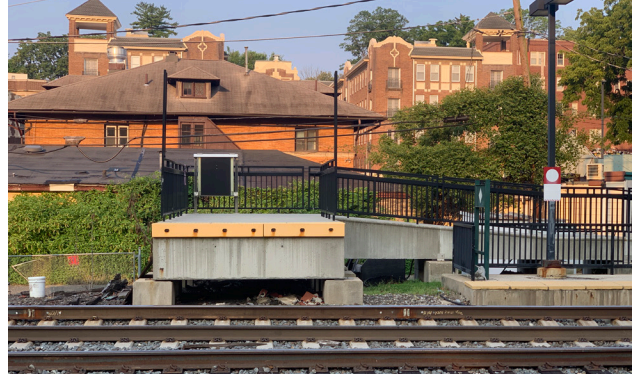
Figure 10: Mini-high platforms allow for level boarding. (DVRPC, 2022)
