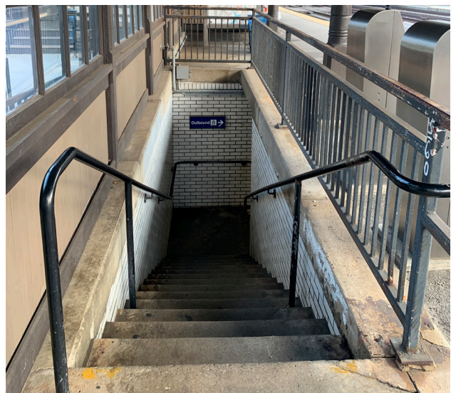
Figure 12: Underpass connecting Regional Rail platforms has stairs on both ends. (DVRPC, 2022)
