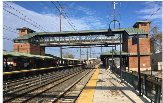
Figure 20: Levittown Station Overpass. Constructed in 2019 over quadtracked Amtrak right-of-way. (Wikimedia Commons, 2019)
