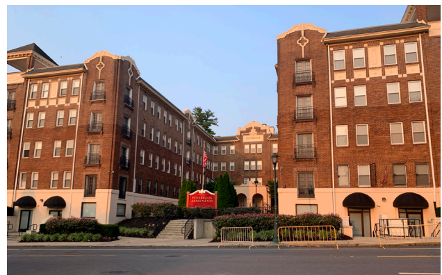
Figure 16: 2134 North 63rd Street, west of Overbrook Station. (DVRPC, 2022)
