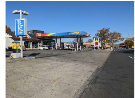
Large curb cuts like those found at the gas station at Broad Street and Hunting Park Avenue create potential conflict points.
