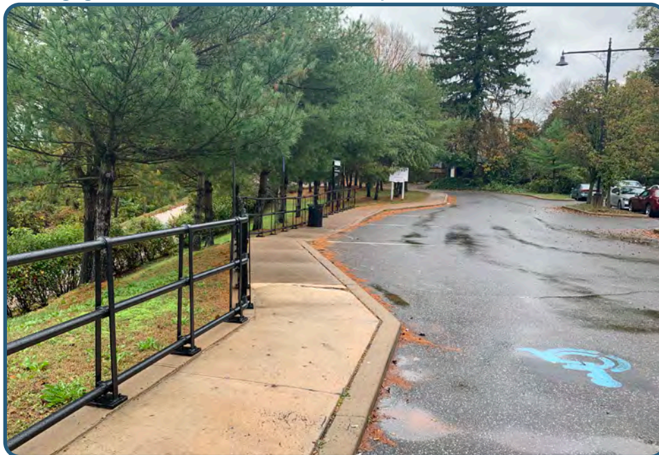
Existing light fixtures at the station, oriented away from sidewalk
