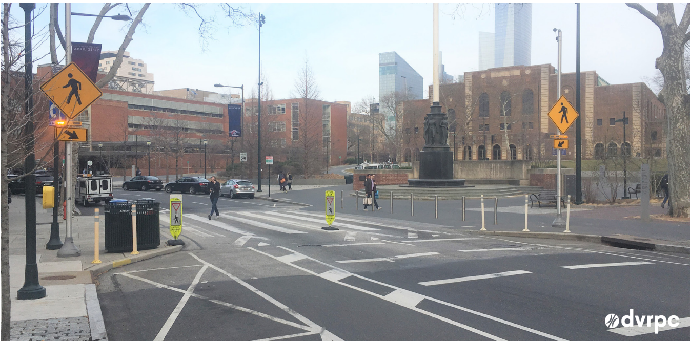
A mid-block crossing with traffic calming elements in Philadelphia.
