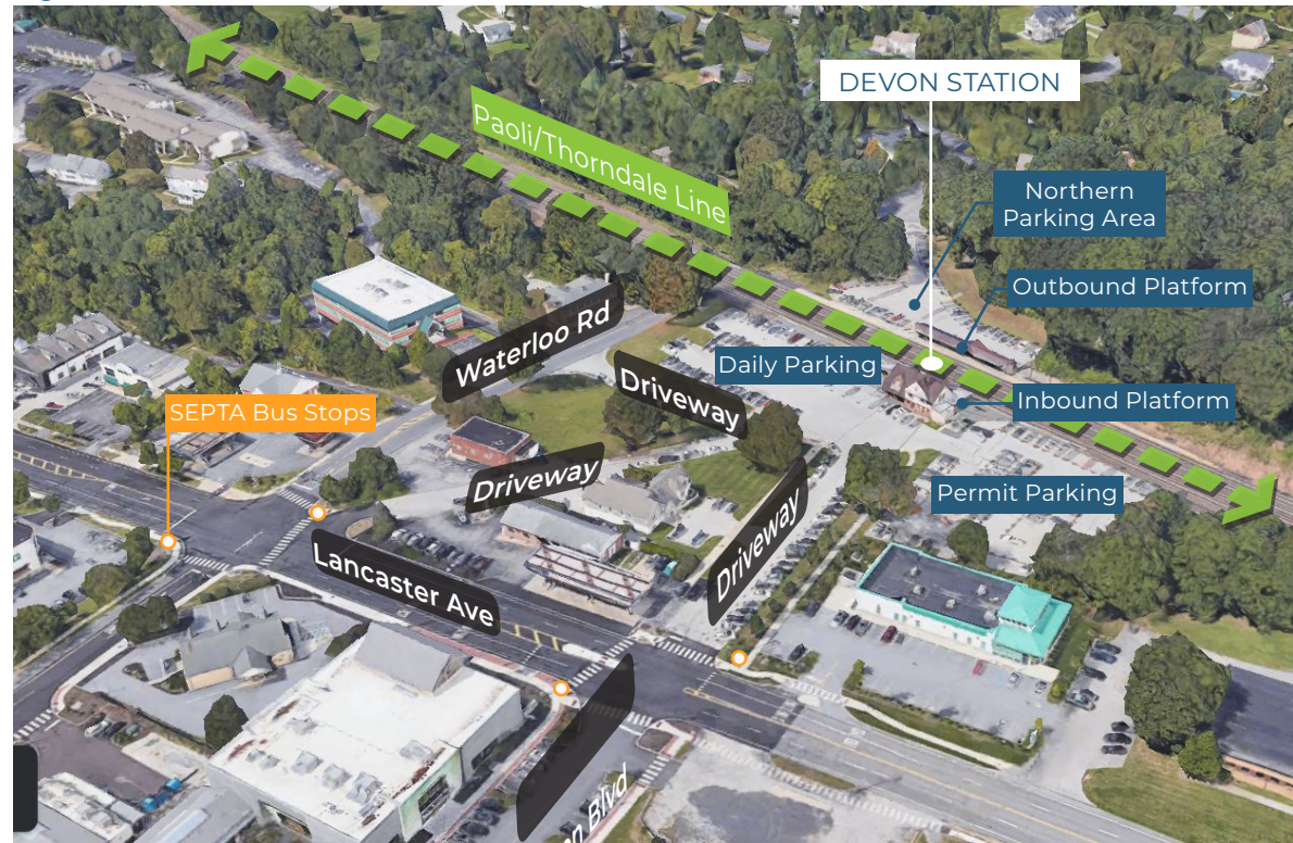
Figure 5: Aerial View of Devon Station
