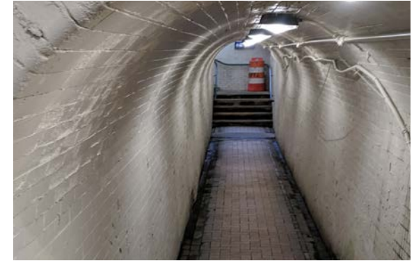
An underground tunnel connects the inbound and outbound platforms.
