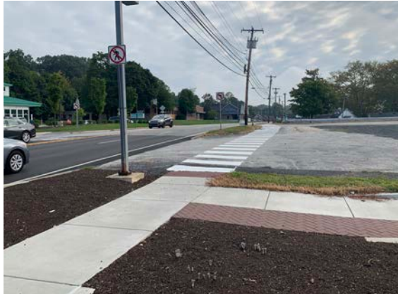
The sidewalk network on Lancaster Avenue is incomplete, and vacant properties inhibit a sense of place.
