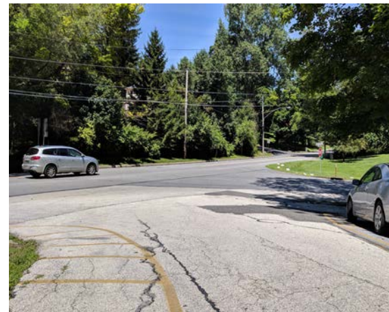
Focus Area 2, N. Waterloo Road, includes a complex intersection that presents challenges and safety issues for all modes.
