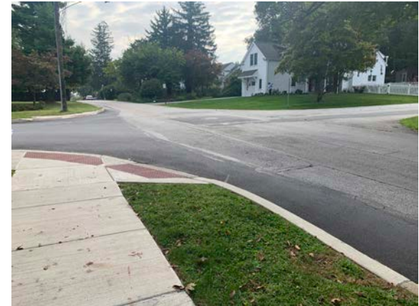
Berkley Road has some sidewalks with curb ramps as shown in the bottom of the frame, although it lacks crosswalks entirely. Furthermore, if a pedestrian crosses in any direction from this corner, they will have to continue their journey in the street.
