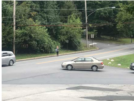
The intersection is complex, lacks a clear hierarchy, and has no safe pedestrian or bicycle facilities.
