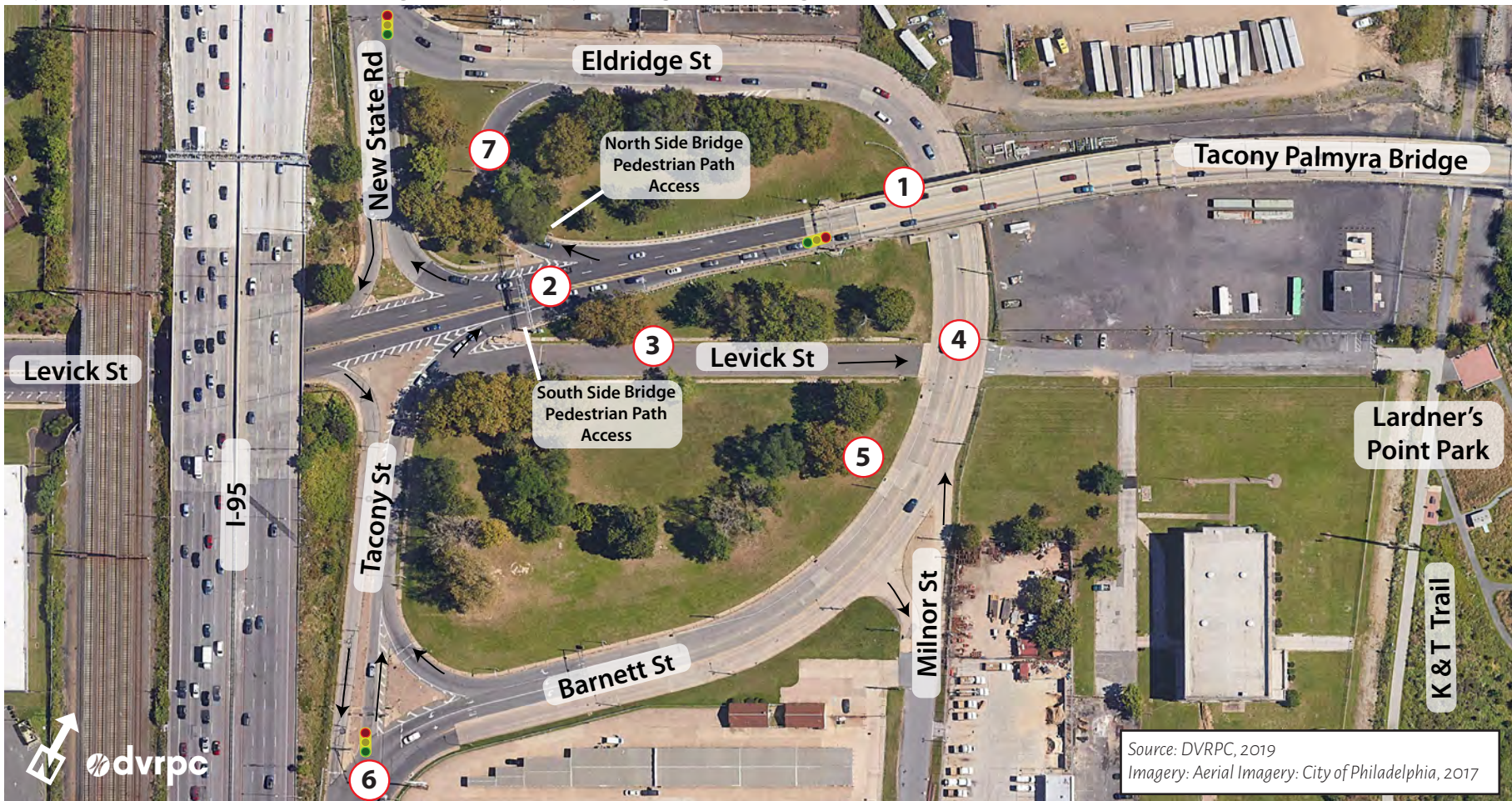
Figure 22 | City of Philadelphia Case Study Issues, East of Interstate 95
