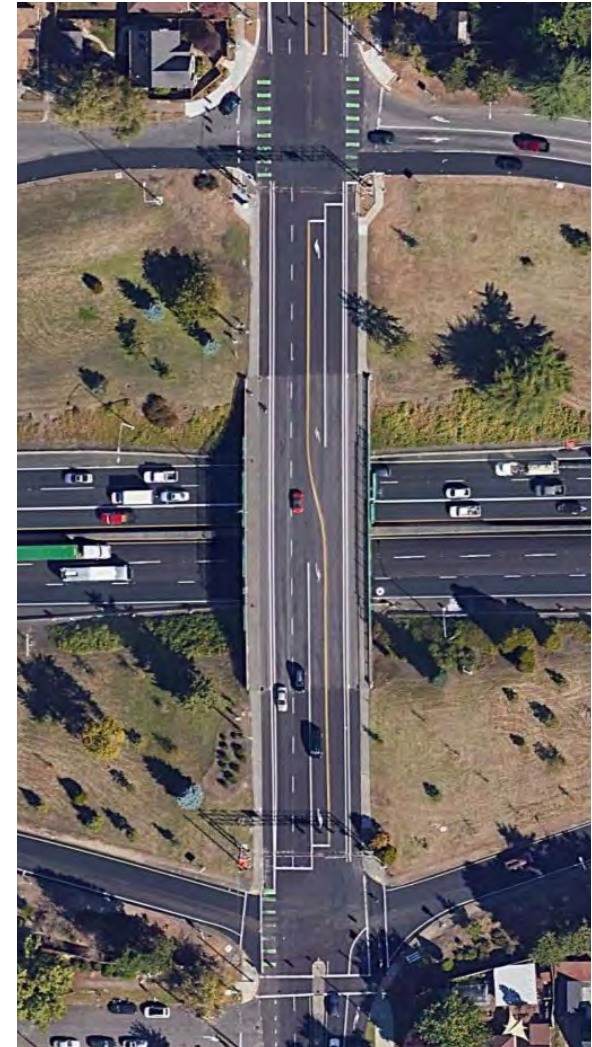
The I-5 interchange at N. Rosa Parks Way in Portland, Oregon, has ramps that meet the intersections at near 90-degree angles, allowing for easier bicycle and pedestrian crossings.
