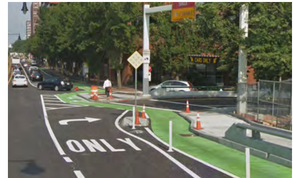
An on-ramp crossing in Cambridge, Massachusetts. Source: Google, 2019
