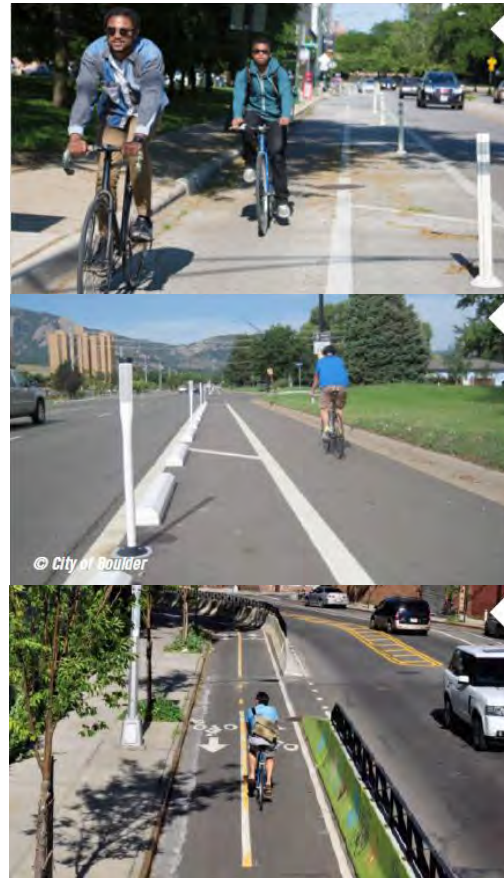
Figure 4 | Low-Cost Interim Solutions for Separated Bicycle Lanes
