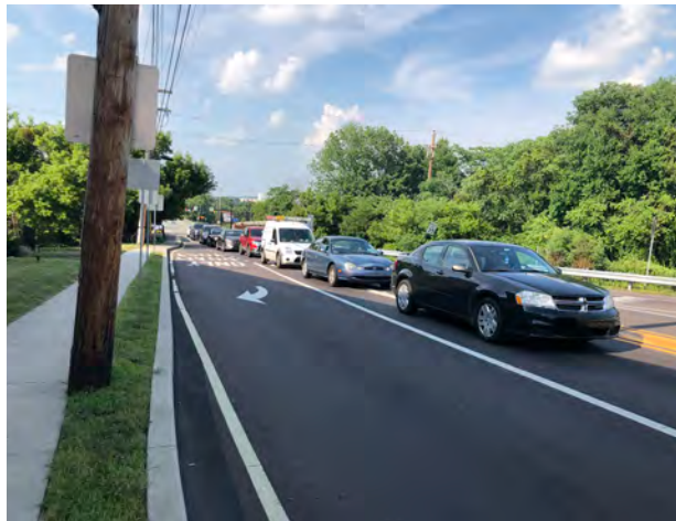
Queueing on SB approach during the PM peak hour. SB through vehicles block the empty right-turn lane. Source: DVRPC, 2018
