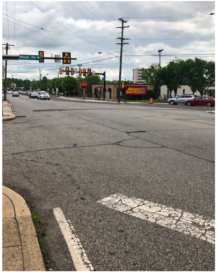
The intersection of High St and Moser Rd is 200-feet-wide. Source: DVRPC, 2018
