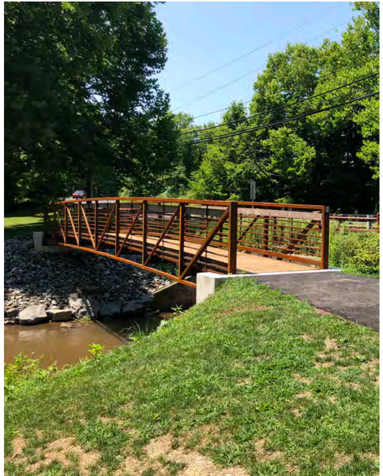
Pedestrian bridge in Murgia Park. Source: DVRPC, 2018
