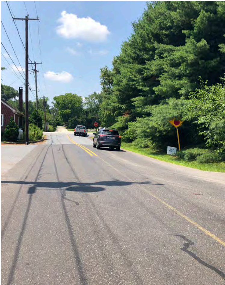
Existing conditions on SB approach of Wells Rd. Source: DVRPC, 2018
