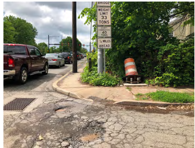
Most of the sidewalk and curb ramps along Armand Hammer Blvd are not ADA-compliant. Source: DVRPC, 2018
