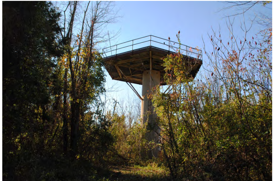
Figure 60: Radar Tower at Former NIKE Site
