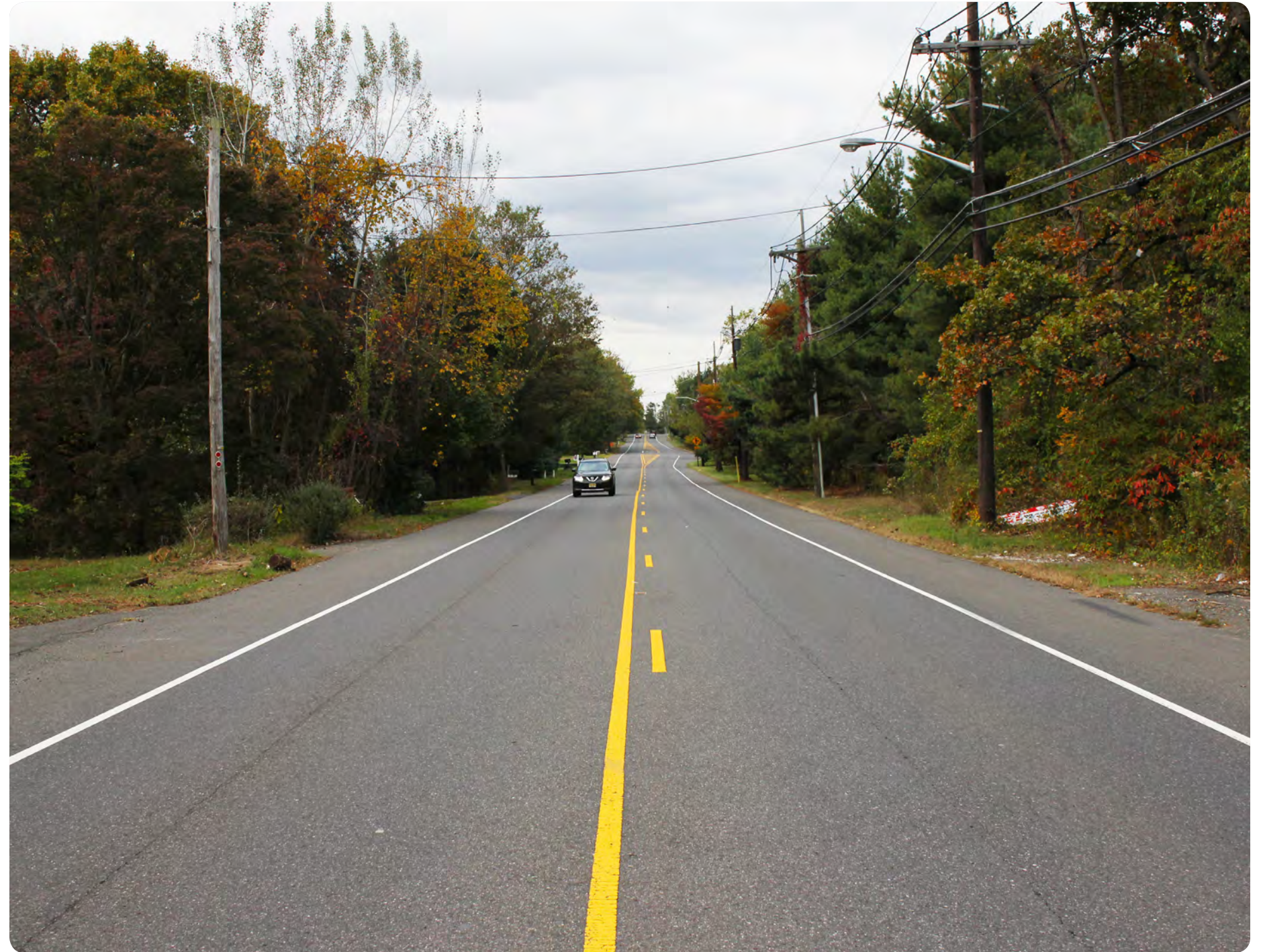
Church Street (CR 607) between Arianas Court and Country Club Parkway is a Minor Arterial in the Urban Area. Based on the estimated existing and future V/C ratio for this segment, the Highway Master Plan recommends current roadway capacity be maintained. Source: DVRPC, 2017
