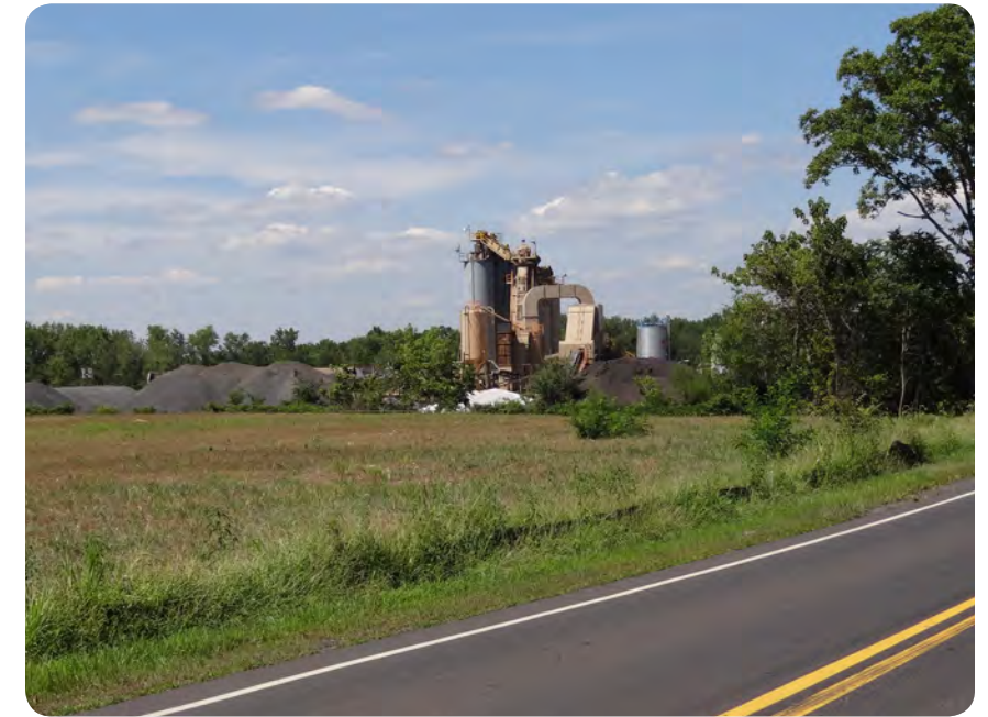
American Asphalt Company manufacturing plant on River Road in Burlington Township. Source: DVRPC, 2016
