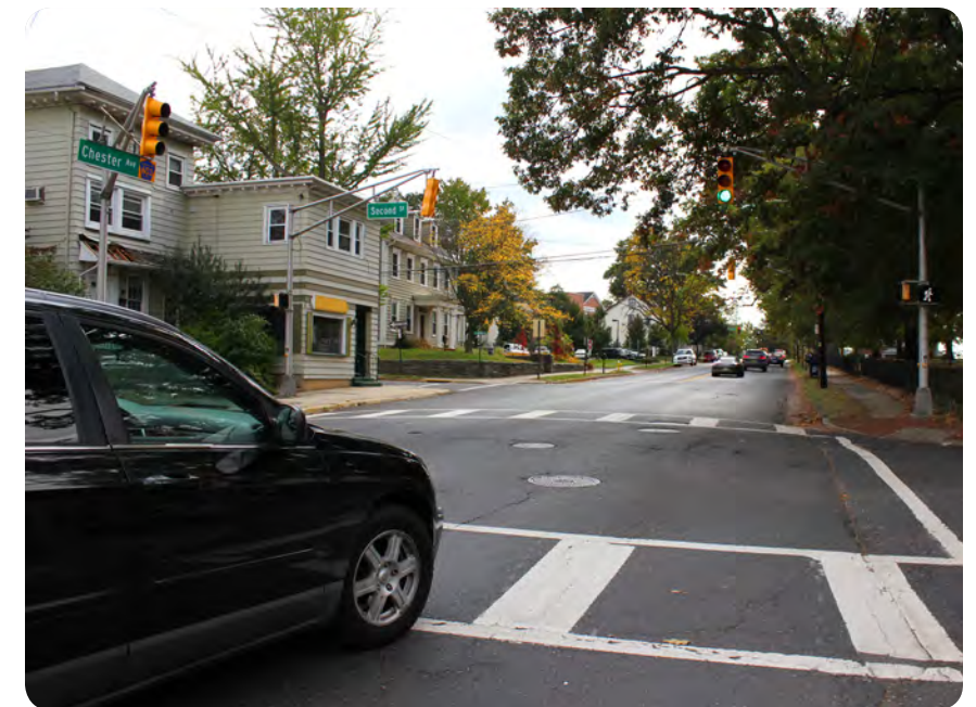
Pedestrian facilities at the intersection of Chester Avenue (CR 603) and Second Street in Moorestown. Source: DVRPC, 2017
