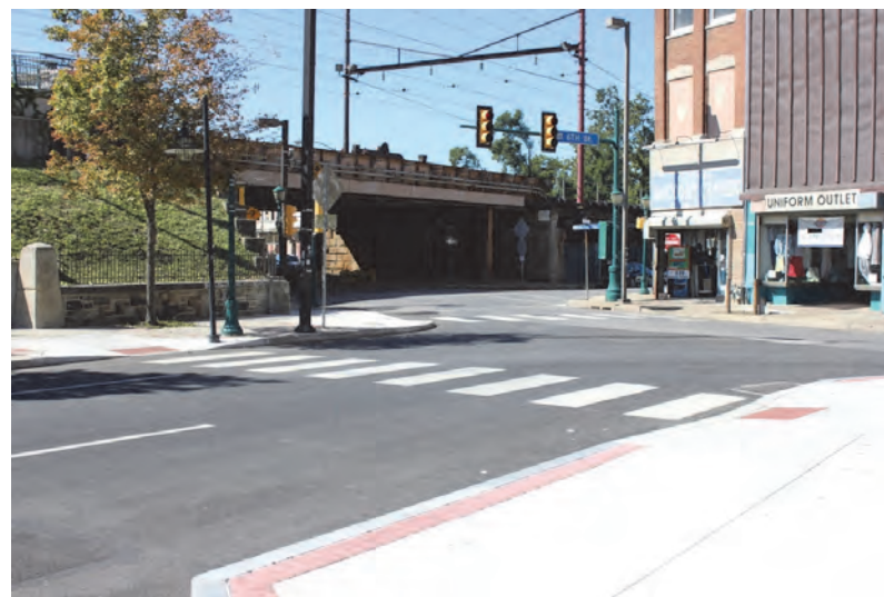
Recent improvements to Welsh Street and 6th Street near the Chester Transportation Center include ADA-compliant curb ramps, sidewalk bump-outs, and highly visible crosswalks. Source: DVRPC, 2017
