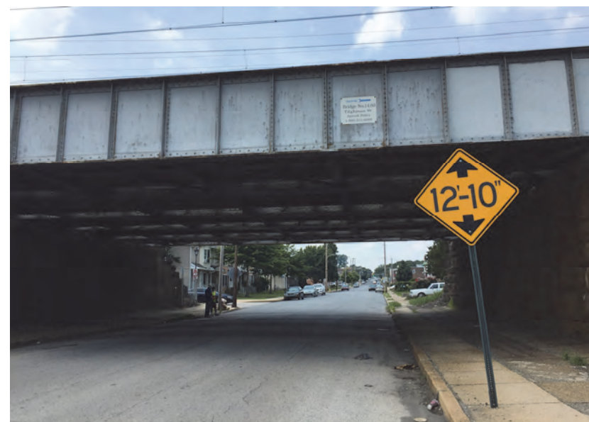
Above: On-bridge clearance signs at Booth Street do not meet PennDOT Publication 236 design guidelines. Source: DVRPC, 2017
