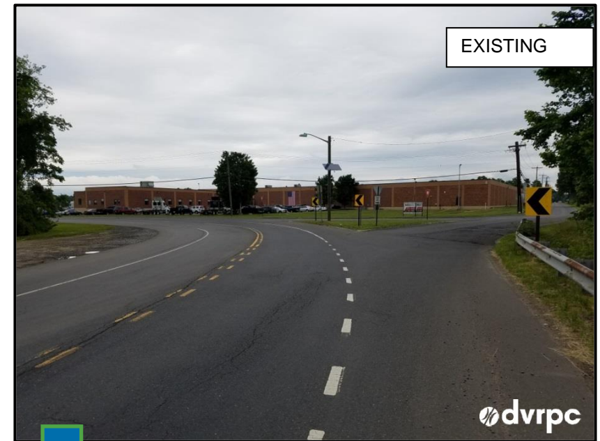
Figure 30: Roundabout at Cedar Lane & Railroad Avenue
