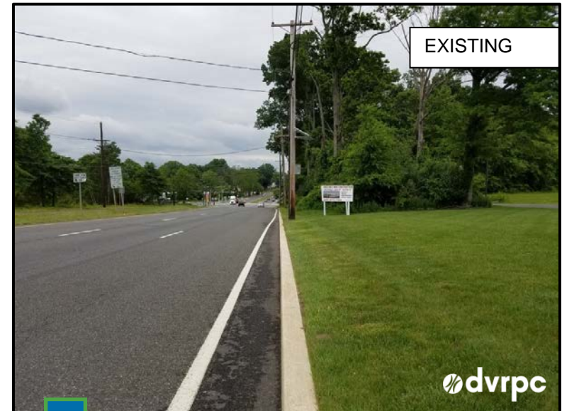
Figure 41: Sidewalk along US 130 from Fairbrook Drive to Hornberger Avenue
