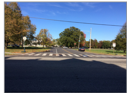
Figure 27: Missing sidewalk connection between Parkside Avenue and PTM
