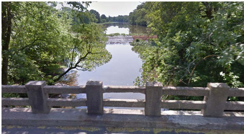
Figure 8: A View of Strawbridge Lake Dam from Kings Highway
