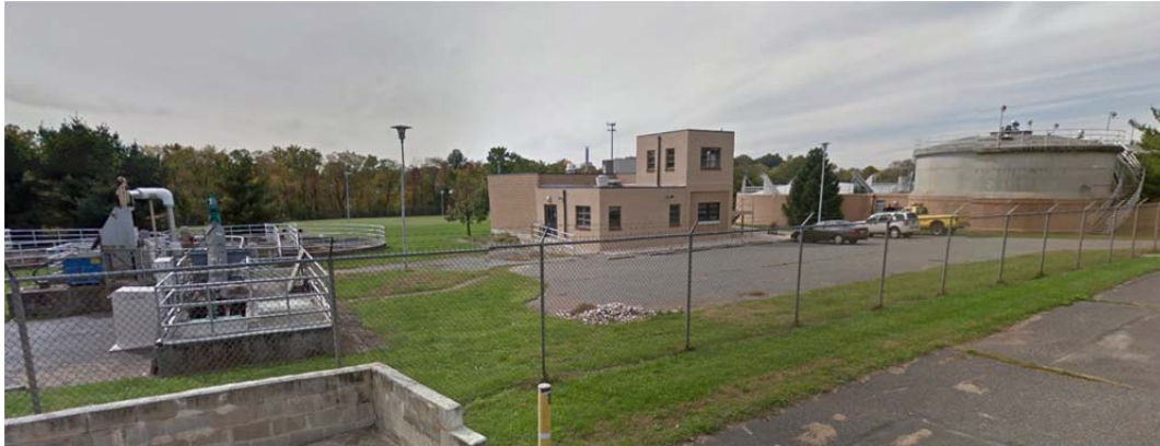
Figure 7: Moorestown Sewer Water Treatment Plant
