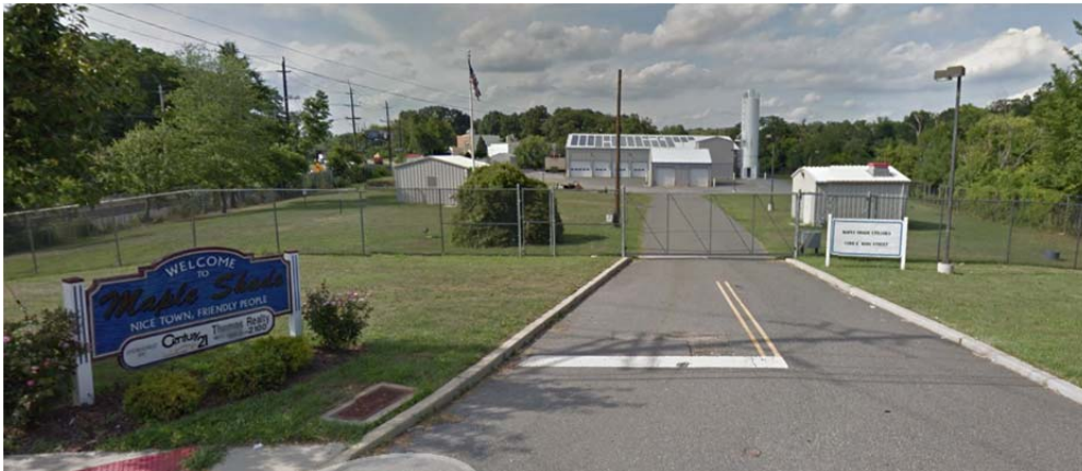
Figure 5: Main Street Pumping Station Site
