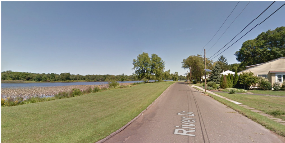
Figure 3: Berm between Rancocas Creek and River Drive, Facing East
