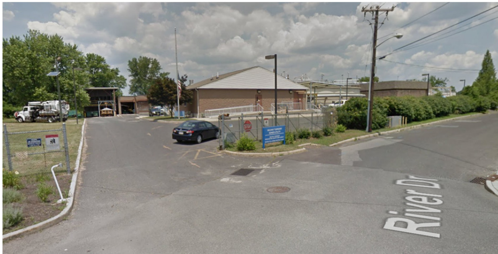
Figure 7: Wastewater Treatment Plant
