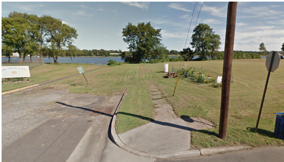
Figure 7: Storm Drain at Penn and Magnolia Streets
