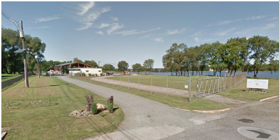
Figure 4: Beverly City Wastewater Treatment Facility
