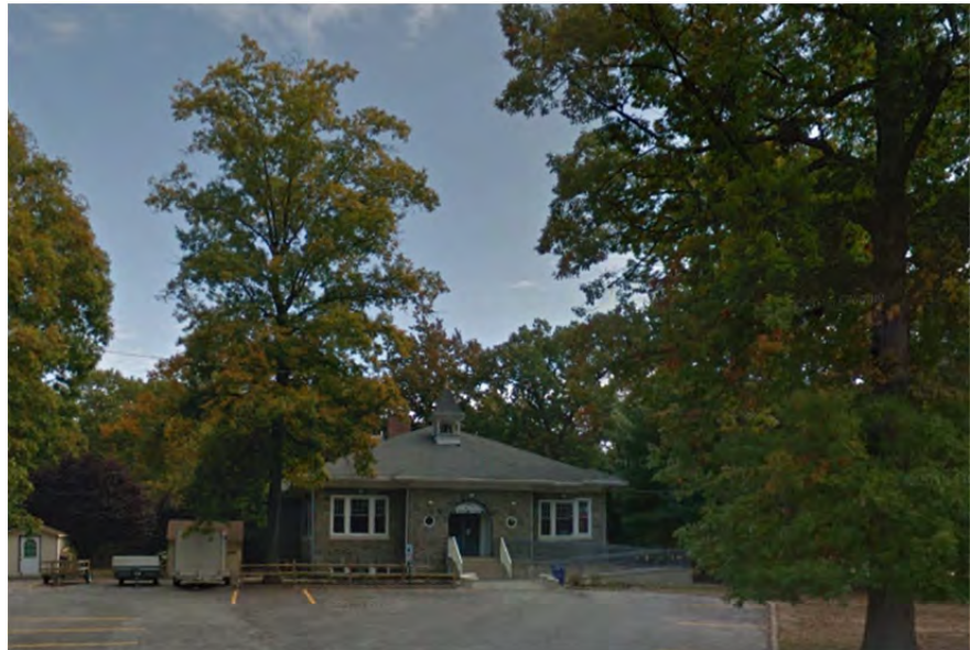
Figure 44: Former Red Bank School No. 1
