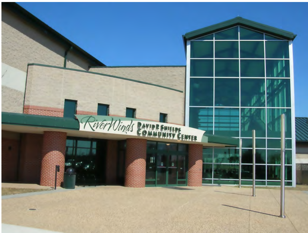
Figure 47: RiverWinds Community Center
