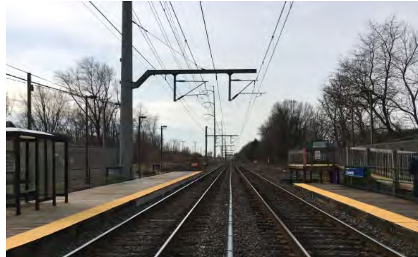
Bi-directional, shared passenger/freight rail track at the Eastwick Station.
