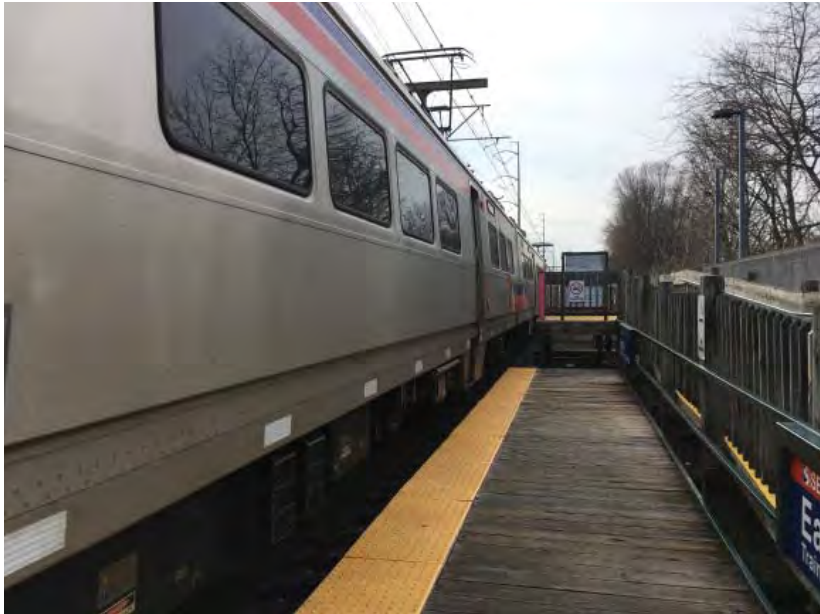
Existing mini-high platform boarding at Eastwick Station.
