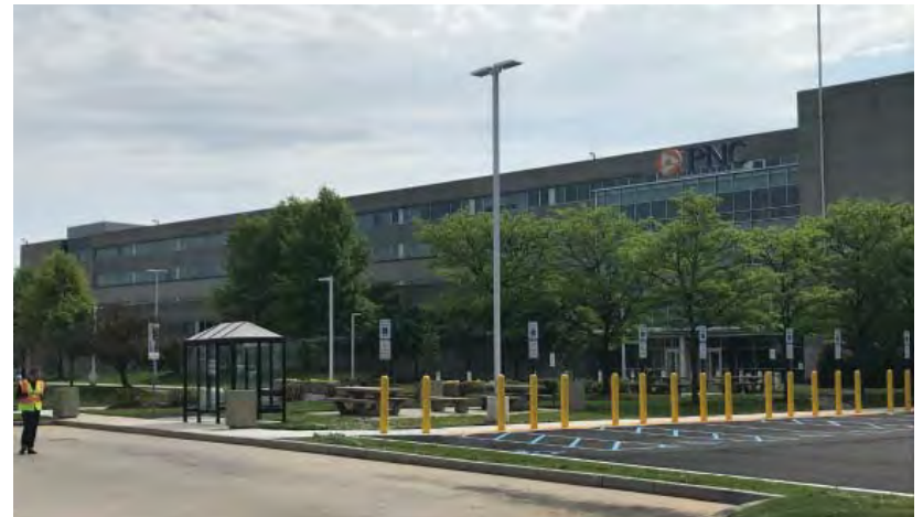
PNC Bank’s Eastwick Center on Tinicum Boulevard.
