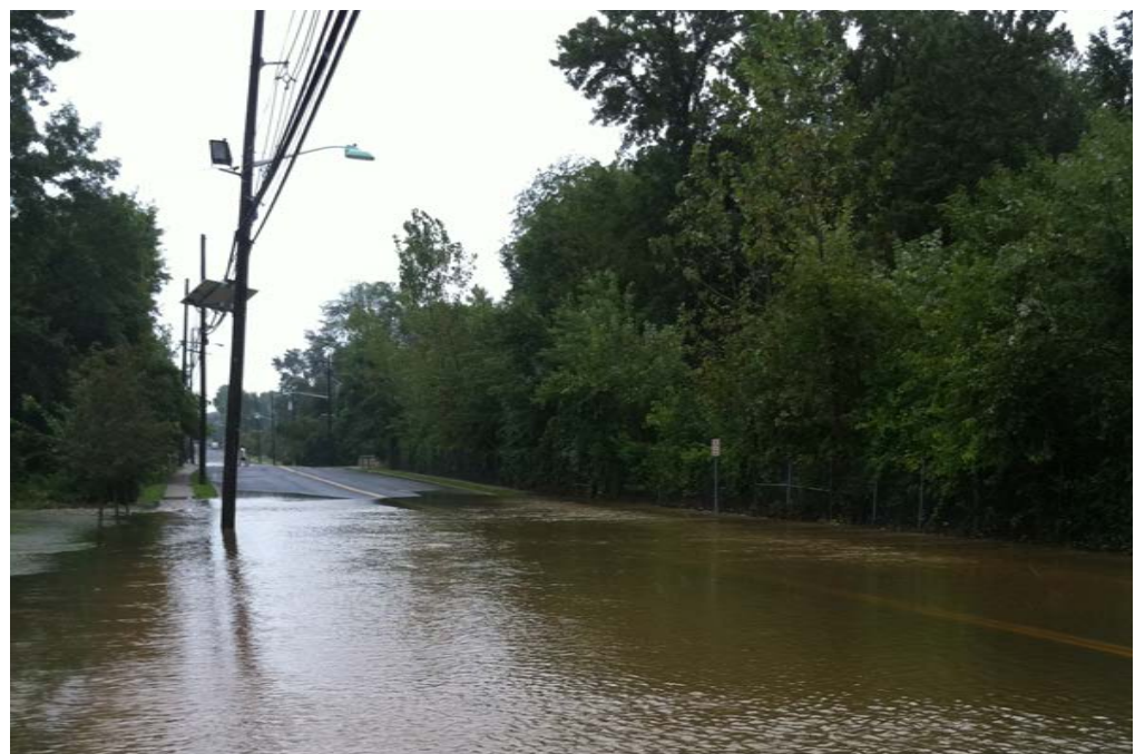
Flooding from Hurricane Irene
