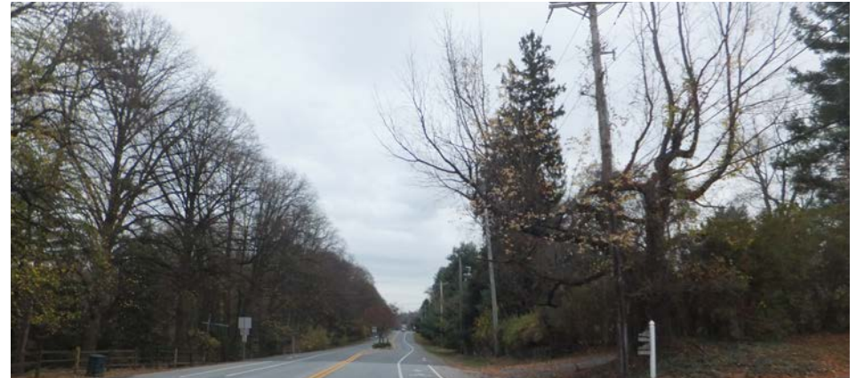
Figure 1.1: Photos of Southern Chester County
