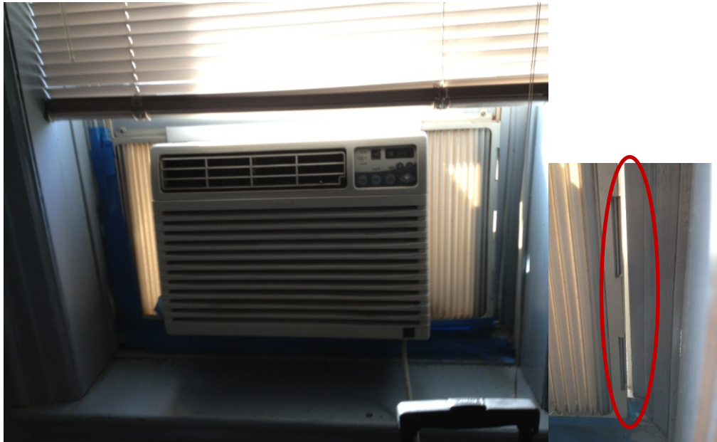
Figure 5: Window Air Conditioner, With Infiltration
