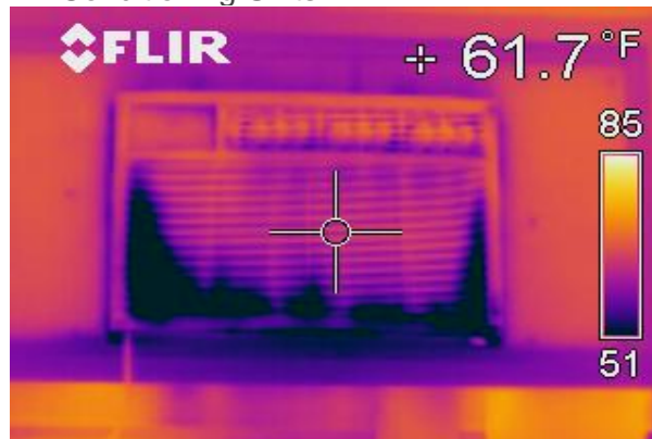
Figure 2: Cold Air Infiltrating Through Window Air-Conditioning Units
