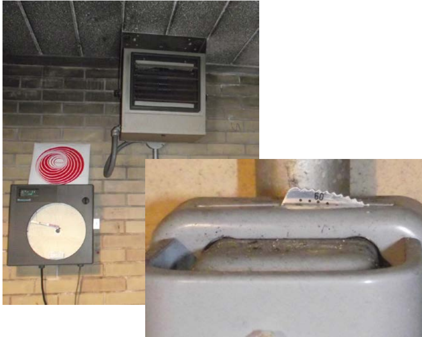
Figure 10: Ground-Level Unit Heater, with low thumbwheel setting
