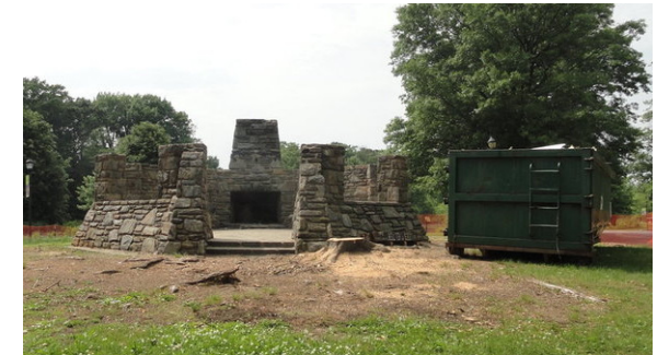
Lees shelter during roof replacement in 2014 Photo Credit: Matt Skoufalos, 2014
