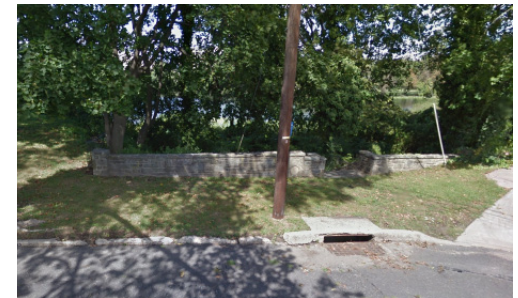
A segment of sidewalk is missing along the north side of Lakeview Avenue near the stair entrance to the park Photo Credit: Google Maps, 2012
