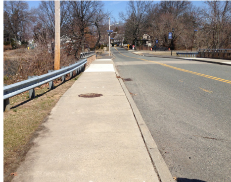
Battlewood Avenue looking north Photo Credits: DVRPC, 2015
