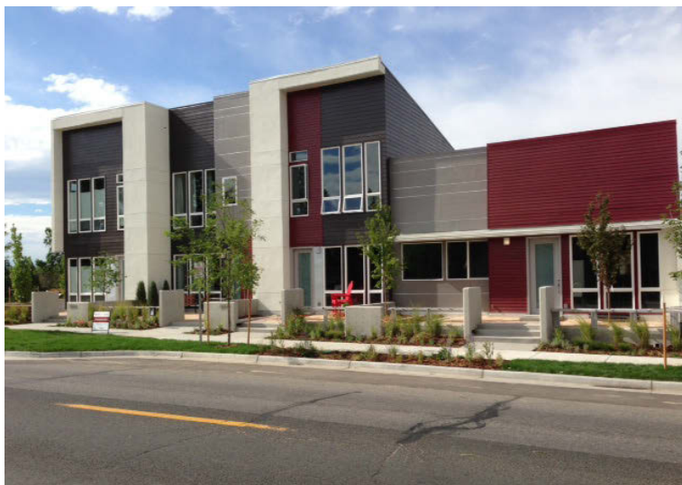
Photo courtesy of Denver Infill
