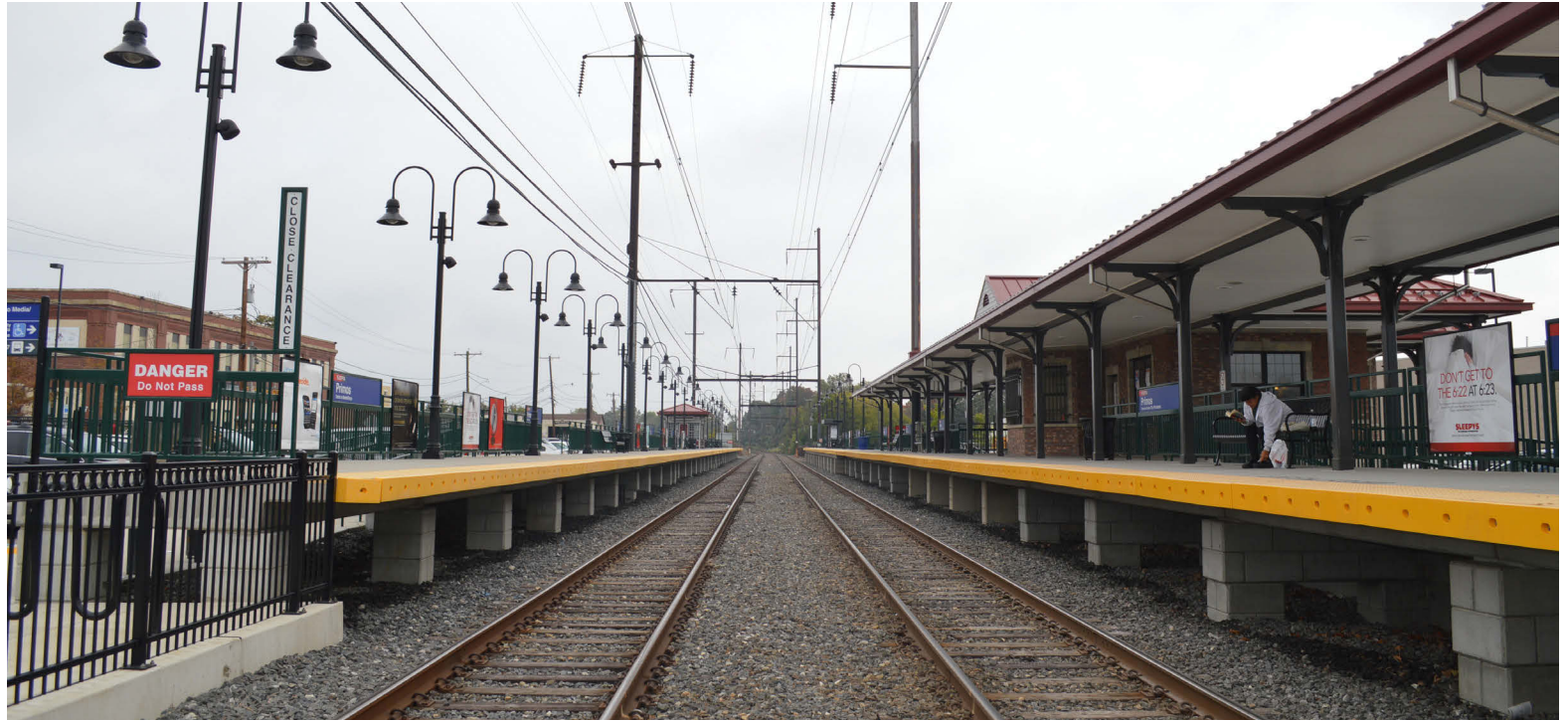
FIGURE 2.5 | Primos Station Image. 2013 Primos Station improvements; high-level platforms were installed for easier and safer boardings. DVRPC, 2014
