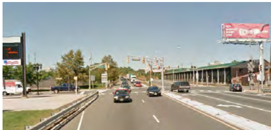
NJ 129 facing north
