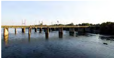
Trenton Morrisville Route 1 Toll Bridge
