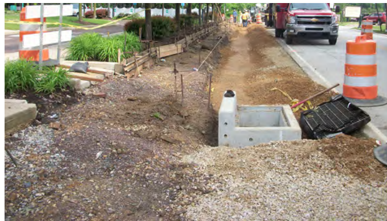
Pedestrian improvements under construction on Bala Avenue in Lower Merion Township, PA Photo Credit: DVRPC
