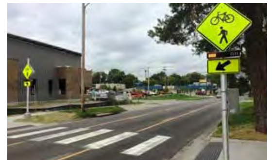
Rapid flashing beacon that is activated by a bicyclist or pedestrian before crossing Photo Credit: City of Lincoln, NE
