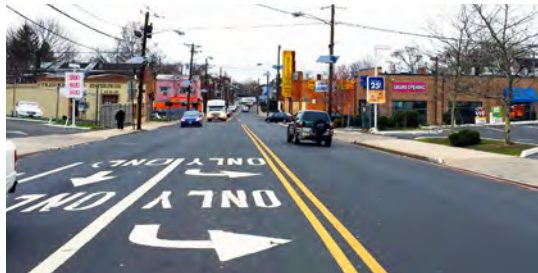
Greenwood Avenue facing west
