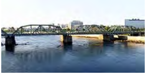
Lower Trenton (Trenton Makes) Bridge
