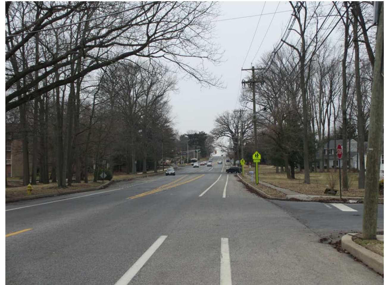
Bike lanes on Somerdale Road (County Route 678) in Voorhees Township are pictured. Camden County's Complete Street Policy will ensure that all modes of travel are considered in engineering, design, and construction of physical improvements to the county route system. (Photo: DVRPC)
