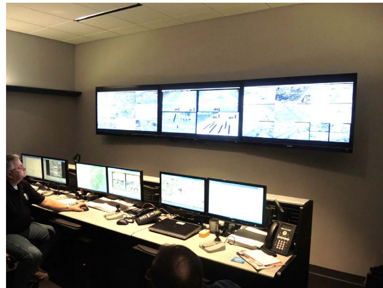
Traffic personnel in the Burlington County Traffic Operations Center, in Mount Laurel, New Jersey, are able to monitor 282 intersections and adjust signal timing at 112 intersections to respond to or regulate traffic flow along their county route system. Similar traffic signal systems are recommended for the Camden County route network. (Photo: DVRPC)
