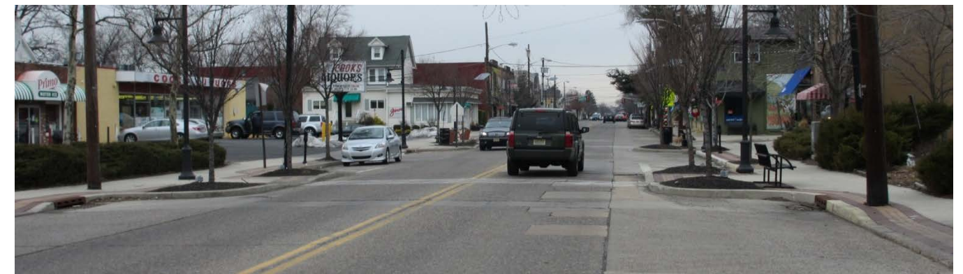
Bulb-outs along Haddon Avenue (County Route 561) in Westmont reduce pedestrian crossing distances. They are proposed at corner bus stops along Broadway (County Route 551) and Federal Street/Market Street (County Route 537)—major bus streets in Camden—to promote NJTransit bus operations and favor its riders. (Photo: DVRPC)
