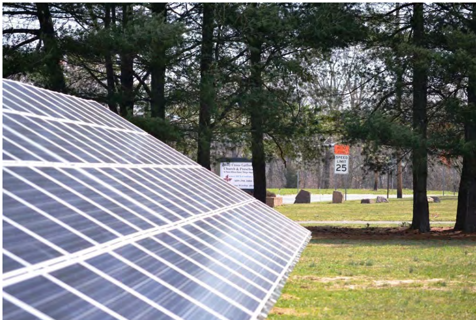
First ground-mounted solar panels
