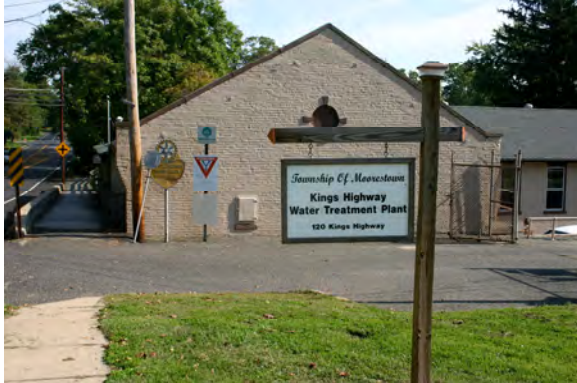
Kings Highway Water Treatment Plant Source: DVRPC
