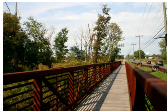
Bridge over Swede Run
