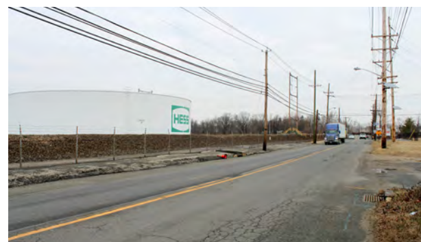
The Hess oil terminal and storage facility is located directly west of PTC.
