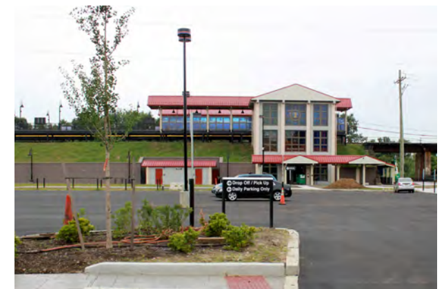
The Pennsauken Transit Center under construction in August 2013.
