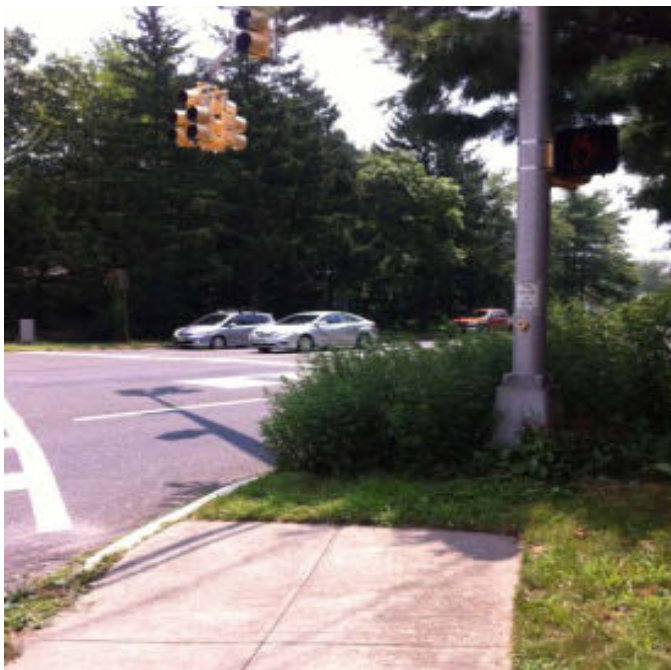
Missing pedestrian connection, overgrown goat path.
