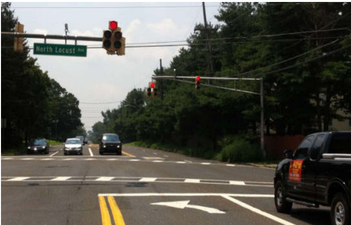
Looking southbound on North Maple Avenue from north side of the intersection; signal head not centered over left-turn lane
