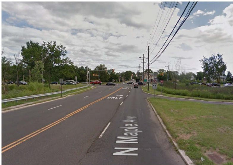
Southbound where the left lane becomes the left-turn-only lane and NJ 70 westbound off-ramp traffic enters North Maple Avenue southbound
