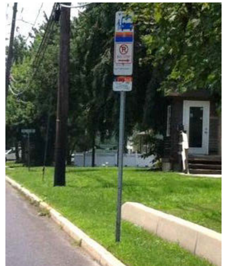
Missing pedestrian accommodations at/to bus stop along corridor northbound
