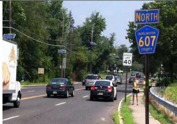
Roadway signs lack retro-reflectivity
