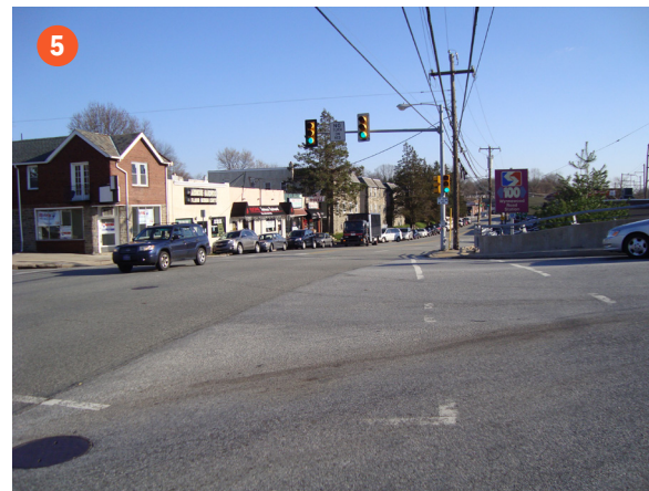
5 Crosswalks at the intersection of Haverford Road and Wynnewood Road/Eagle Road need to be repainted.
