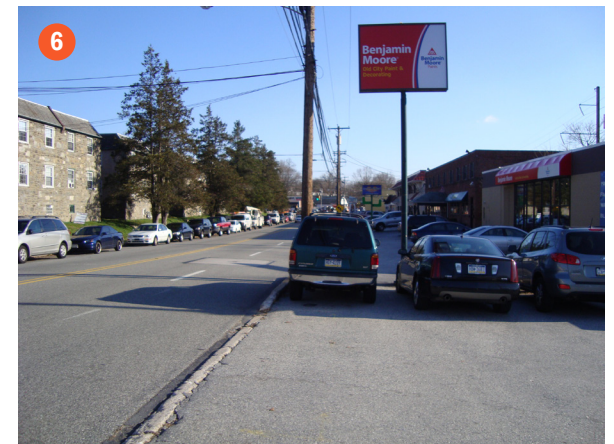
6 Cars parked at the Wynnewood Road Station obstruct pedestrians.
