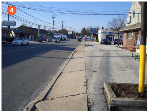
4 In many places, sidewalks rise and fall at parking lot access points creating potential hazards for pedestrians.
