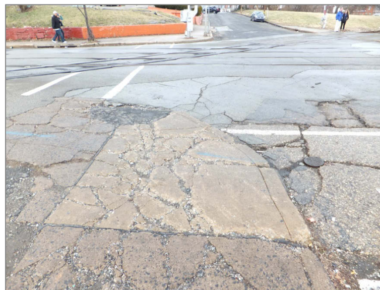
Figure 4: Existing sidewalk conditions at Main and Sixth streets crossing
