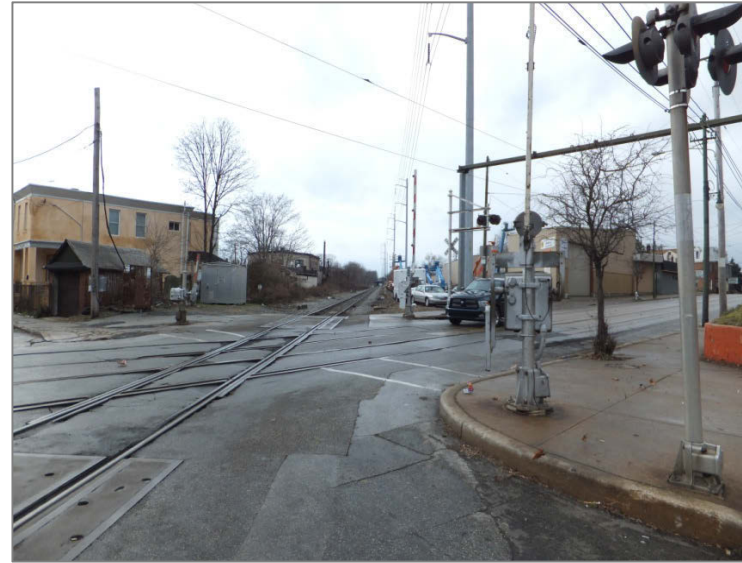
Figure 2: Pavement degradation at the Main and Sixth street crossing, concentrated around rail flanges
