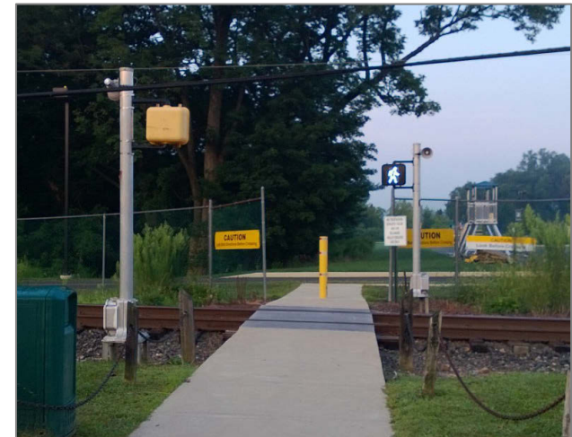
Figure 6: Example of a pedestrian signal at a grade crossing, Delaware Valley College, New Britain, PA Source: DVRPC
