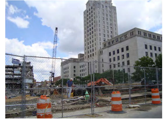
Work has begun on public space improvements near Camden City Hall.
