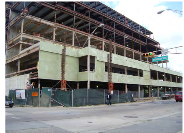
The Cooper Medical School of Rowan University is currently under construction along Broadway between Benson Street and Washington Street.
