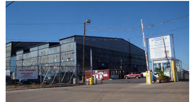
A variety of port and industrial uses can be found in the southwest portion of the Ferry Avenue station area.
