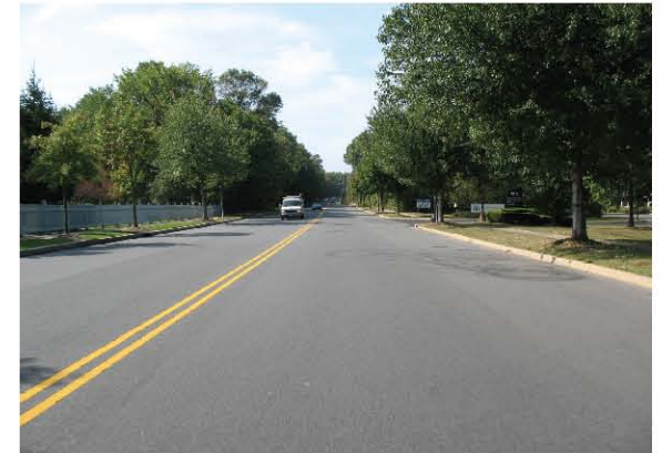
This section of Clarksville Road contains a housing complex (left) and a shopping center (right), but no pedestrian crossing between the two.
