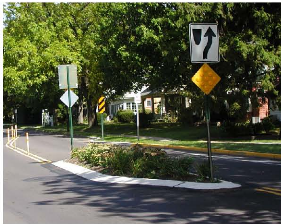
▲ The West Court Street traffic calming project in Doylestown incorporated a number of elements to slow traffic in front of Central Bucks West High School and create a gateway into the borough.
