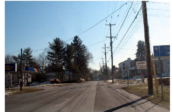
The existing conditions on PA 896, looking south toward the intersection of Appleton Road.
