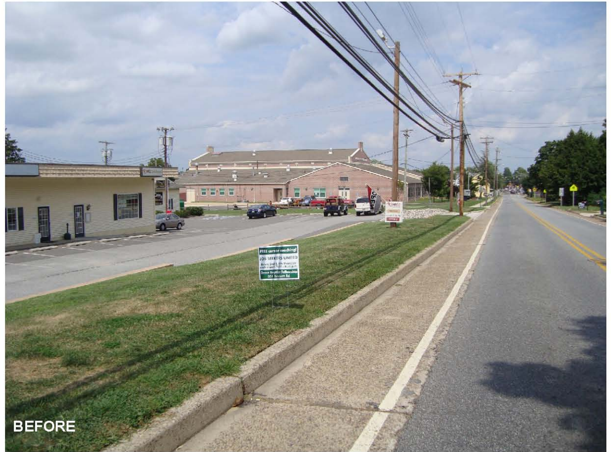
FIGURE 5: CR 551 - EXISTING CONDITIONS
