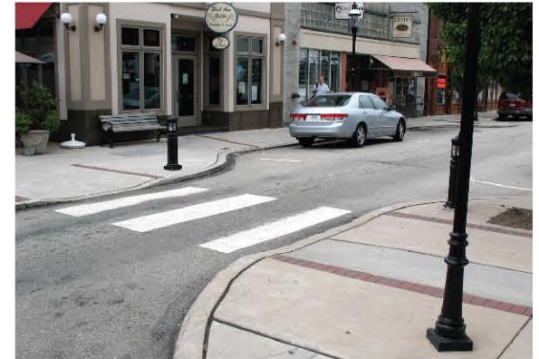
These curb bumpouts in Jenkintown, Pennsylvania, force traffic to slow down, while shortening the pedestrian crossing.
