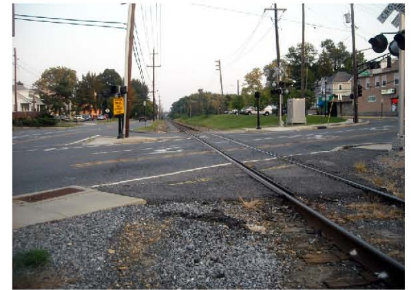
Existing railroad tracks along East Atlantic Avenue near Clements Bridge Road.
