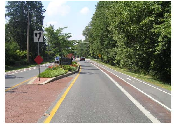
This center island in Centreville, Delaware, narrows travel lanes and acts as a gateway. Special paving is also used to create a safe buffer for cyclists.
