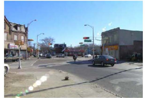
Haddon and Kaighn avenues meet at an oblique angle, resulting in a lengthy pedestrian crossing.
