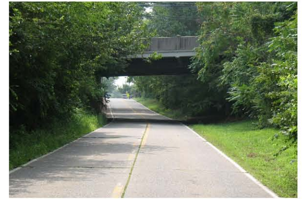
Looking east along East Atlantic Avenue toward Haddon Heights Elementary School.
