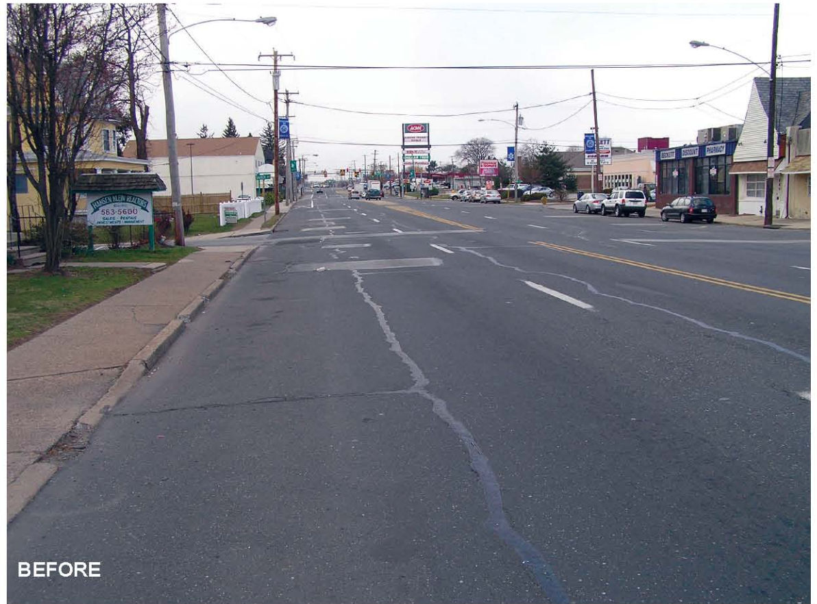
FIGURE 26: CHESTER PIKE - EXISTING CONDITIONS
