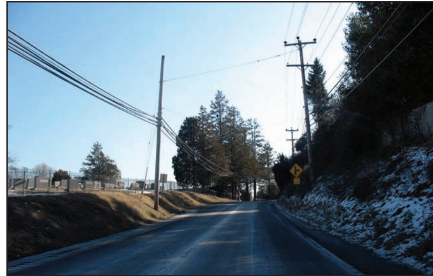
Horizontal and vertical curves, like the one shown here, looking south along PA 896, just past Parsons Road, compromise sight distances. Directly over this curve is the Avon Grove school and the village center. Source: DVRPC
