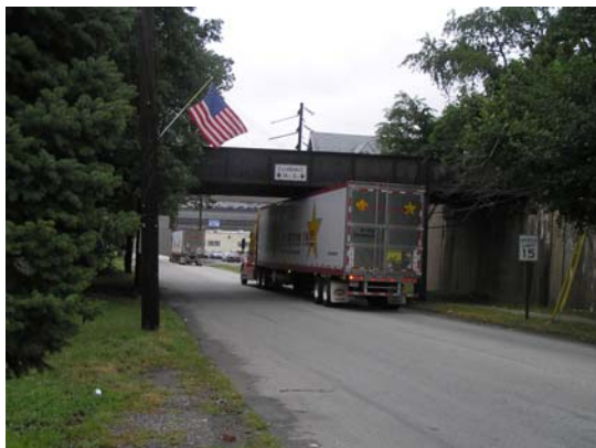
A truck passing under a rail bridge along Saville Avenue entering Penn Terminals.
