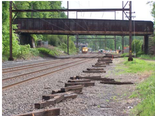
Photograph of a Norfolk Southern railroad track crossing over CSX's Trenton subdivision near the SEPTA Woodbourne, PA, passenger station. (Photograph provided by CSX)
