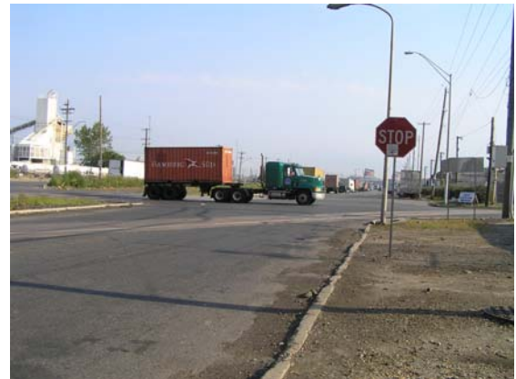
A truck on the NHS Connector for the South Philadelphia Freight Complex (Photo provided by DVRPC)
