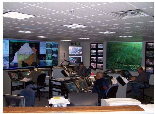
The PennDOT District 6 Traffic Operations Center.
