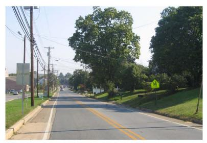
Auburn Avenue's straight alignment and 'in-between' context contribute to excessive vehicle speeds. Source: DVRPC
