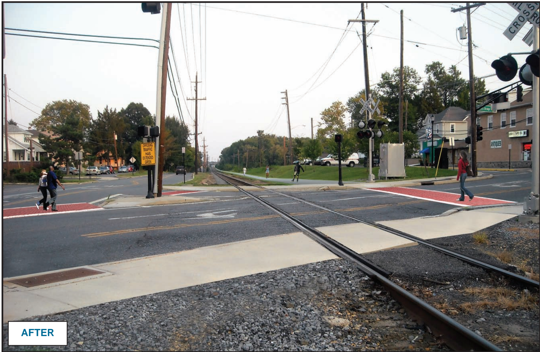
FIGURE 29: Vicinity of Clements Bridge Road, Looking East – Simulation. This image is a photo-simulation of the recommended improvements applied to the location shown on the left. Major improvements include the multi-use trail crossing over to the south-side of the railroad tracks, high-visibility crosswalks, and improved sidewalk treatments. Source: DVRPC
