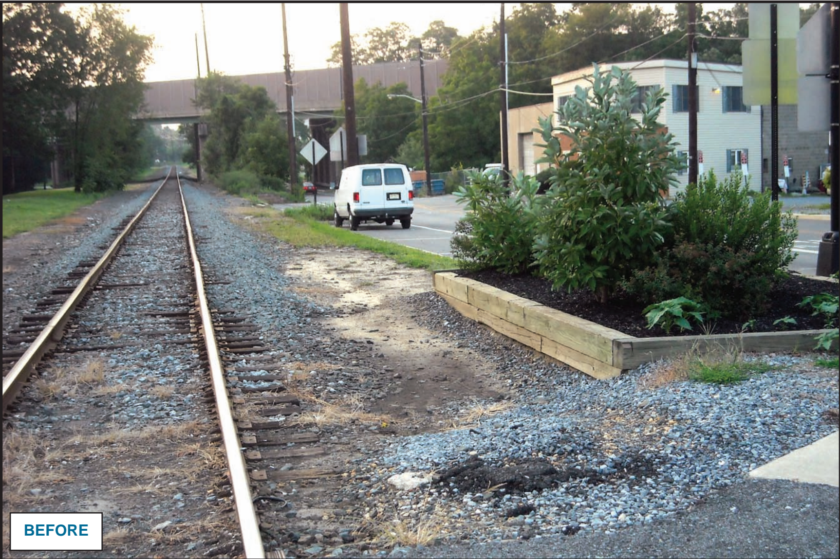
FIGURE 26: Vicinity of Clements Bridge Road, Looking West – Existing Conditions. This image is a photograph of existing conditions by East Atlantic Avenue, looking west. Source: DVRPC
