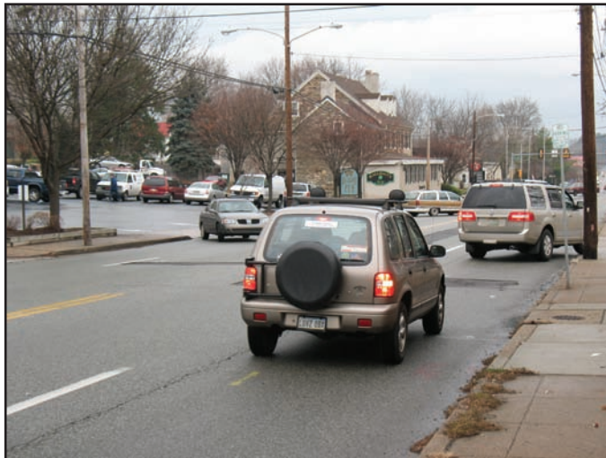
The collection of several, staggered access points by the Acme shopping center creates conflicts between turning and through traffic. Source: DVRPC
