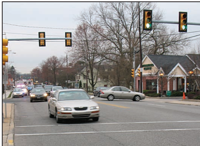
The offset intersection coupled with the Starbucks access point creates a confusing intersection with poor sight lines, and a demonstrated crash history. Source: DVRPC
