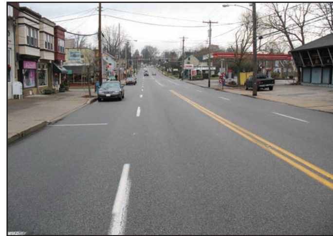
The need for on-street parking and the lack of dedicated parking lanes results in this unusual allowance of on-street parking in an active travel lane — a potentially dangerous condition.
