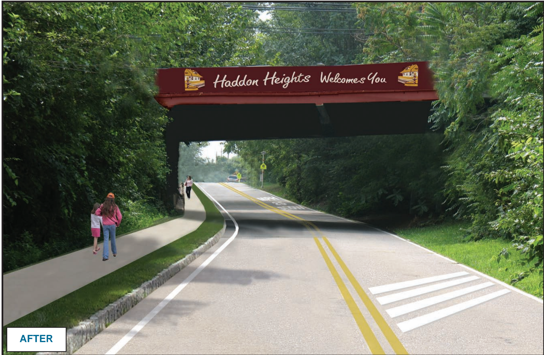
FIGURE 21: Vicinity of Haddon Heights Elementary School – Simulation. This image is a photo-simulation of the recommended improvements applied to the location shown on the left. Major improvements include an increased curve in the roadway to accommodate sidewalks and grass buffer (shown at left), re-striping of the roadway, speed limit pavement markings, and rumble stripes. Source: DVRPC
