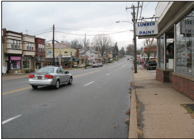
The straightaway past the curve at Gordon Lane (northbound) results in drivers accelerating just as they are entering a traditional business district where high speeds are inappropriate.
