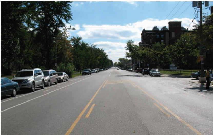
The long straightaway on Parkside Avenue, between 52nd Street and Belmont Avenue, is 3,000 feet without a traffic signal, creating ideal conditions for speeding. Source: DVRPC
