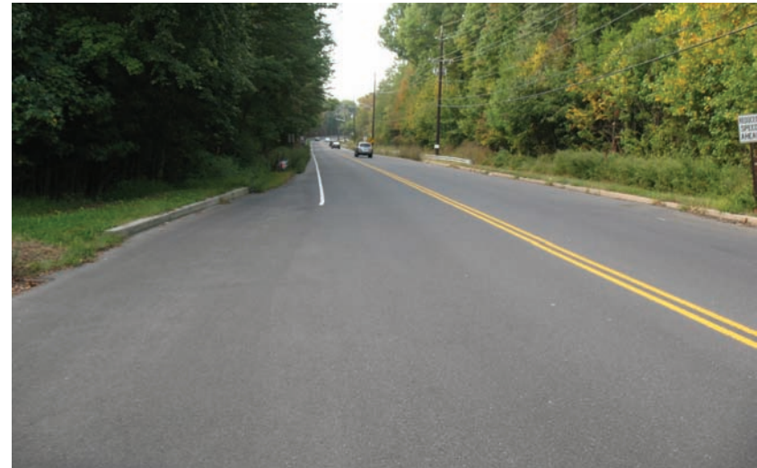
The roadway width changes dramatically and suddenly at various points. This image shows the area just to the south of the Avalon Watch housing complex. Source: DVRPC
