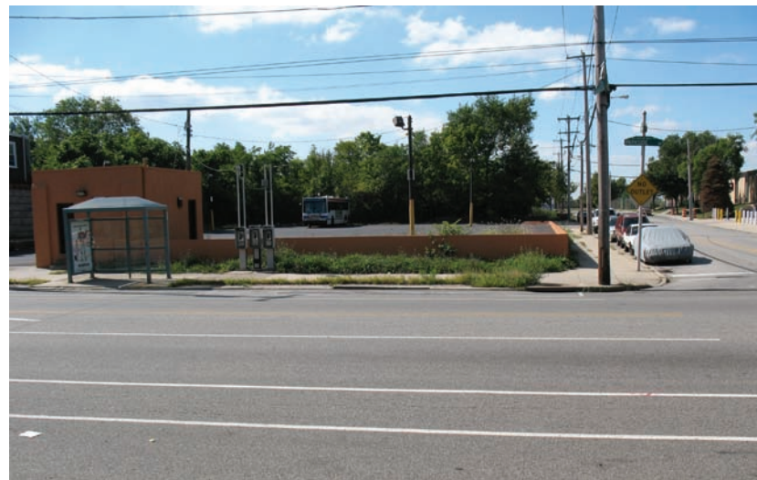
The SEPTA bus terminal at 49th Street (shown above) is unattractive and uninviting. Transit stops throughout the corridor are not well marked and have poor facilities for riders. Source: DVRPC
