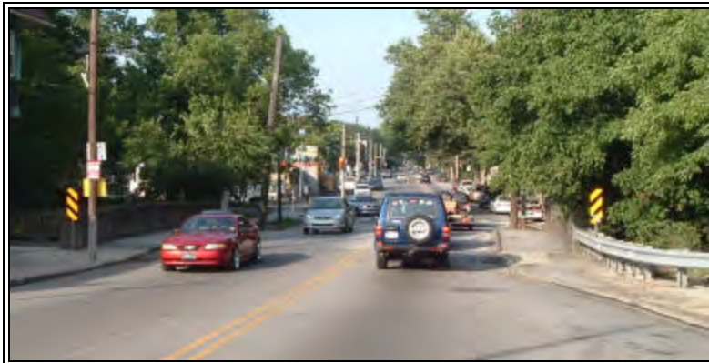
Bridge over Cobbs Creek
