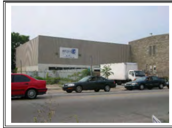
Industrial and commercial uses through Upper Darby (East).
