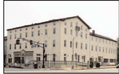
Seniors have more housing options with the addition of the Metropolitan Inn, a mixed-use building including age restricted apartment rentals. Source: DVRPC
