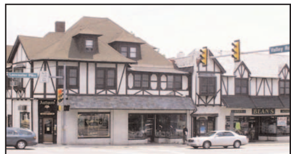
Traditional commercial development adjacent to the Paoli station.
