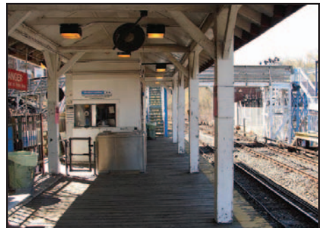
Millbourne Station was once in disrepair but construction to improve and enhance the station is nearly complete.
