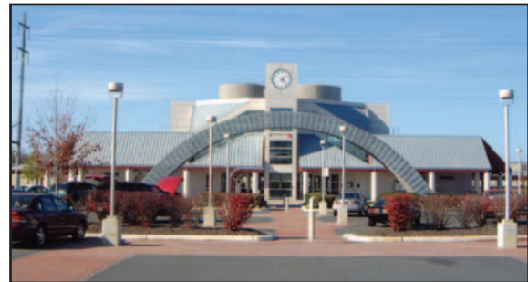
Above: Current Hamilton station may be a part of a larger TOD if the developer can reach an agreement with local officials.
