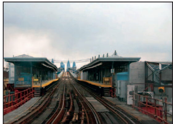
SEPTA is currently renovating 63rd Street station.
