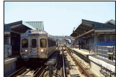
Passengers wait for an El train at recently renovated 56th Street station.
