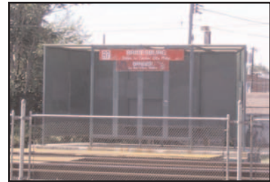
Bridesburg station is currently being studied for possible enhancements and access improvements.
