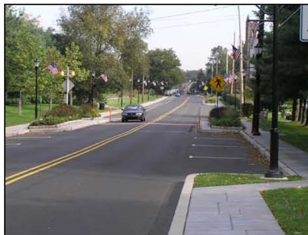
Streetscape improvements recently constructed along Sycamore Street in Newtown Township contain curb extensions and other traffic calming elements Photo by: DVRPC
