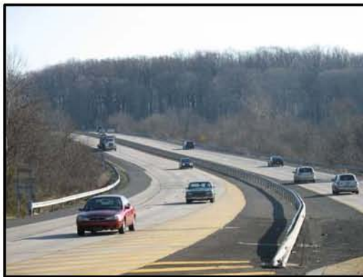
Typical section of the Newtown Bypass Photo by: Jacobs Edwards and Kelcey
