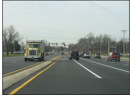
Newtown Bypass at Lindenhurst Road Photo by: Jacobs Edwards and Kelcey
