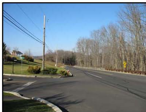
Worthington Mill Road at Lantern Way, looking northbound Photo by: Jacobs Edwards and Kelcey
