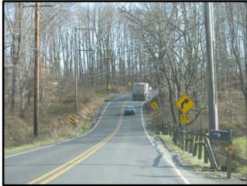
Swamp Road, between Second Street Pike and Worthington Mill Road, looking eastbound Photo by: Jacobs Edwards and Kelcey
