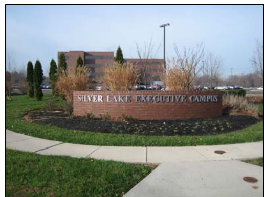
Silver Lake Executive Campus on the Newtown Bypass Photo by: Jacobs Edwards and Kelcey
