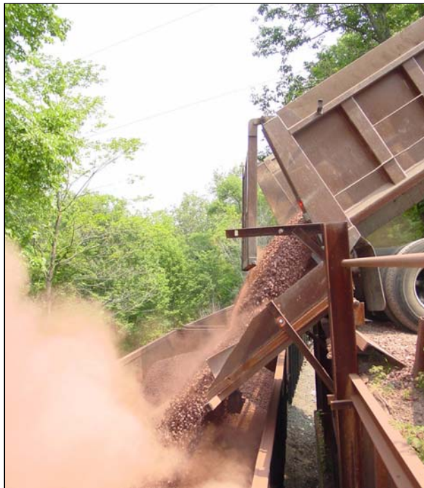
Transloading in operation at the Mill Creek Road rail hub site [note: Wrightstown’s quarries produce “blue” stone. The red stone is from remote quarries—indicative that quarry trucks from outside of Wrightstown are also present on the Key Roadways.]
