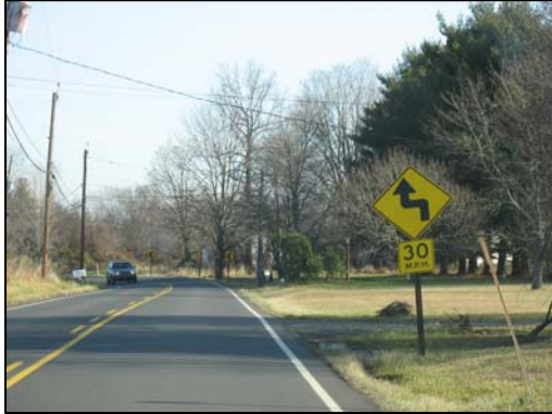
Advisory signs along Wrightstown Road (looking eastbound) near Old Dolington Road Photo by: Jacobs Edwards and Kelcey
