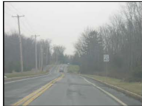
Typical section of Lindenhurst Road Photo by: Jacobs Edwards and Kelcey
