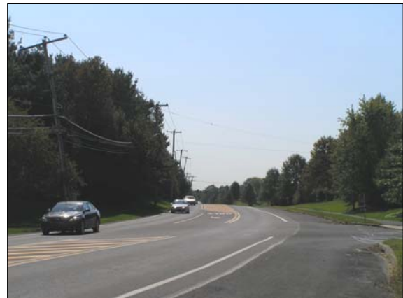
Lindenhurst Road is proposed to include raised median islands, textured cross-walks, and narrowed travel lanes Photo by: DVRPC
