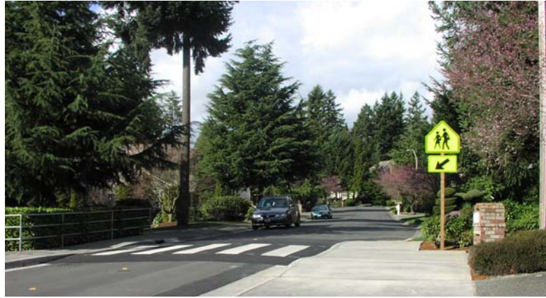
An example of a raised crosswalk is pictured. At this time, PennDOT only considers textured crosswalks on state highways. Photo by: John Carpita, Public Works Consultant, Municipal Research and Services Center of Washington, Spring 2005 Issue
