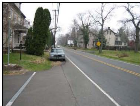
Typical section of Second Street Pike in Wrightstown Township Photo by: Jacobs Edwards and Kelcey
