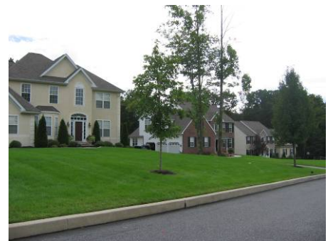
Single-family home construction in Chester Heights Borough (top) and Middletown Township (bottom) continues to bring new residents to the area.
