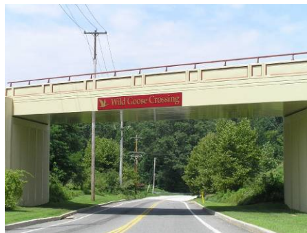
This bridge across Valley Road in Middletown Township links Wawa Dairy Farms' Corporate University and dairy plant.
