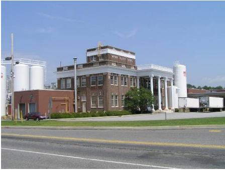
Wawa Dairy's processing and bottling plant, which was built in 1929 at the intersection of Baltimore Pike and Valley Road.
