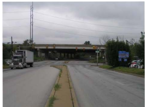
A sign at the Philadelphia International Airport directs users to the NHS routes nearby
