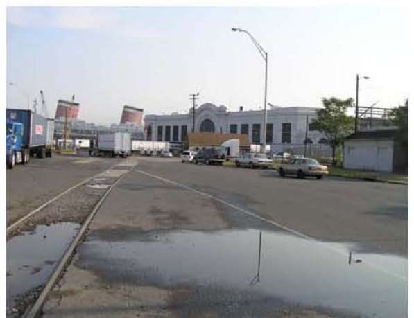
Rail line crosses Old Delaware Ave. to serve Pier 84 along the South Philadelphia Freight Complex connector
