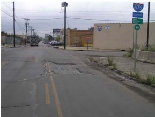
Cobblestones show through the street on the Beckett Street Terminal Connector
