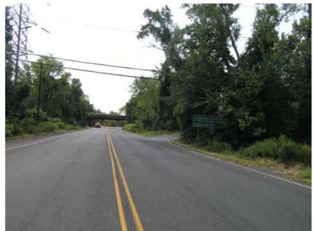
A newly paved road on the Port of Bucks Connector
