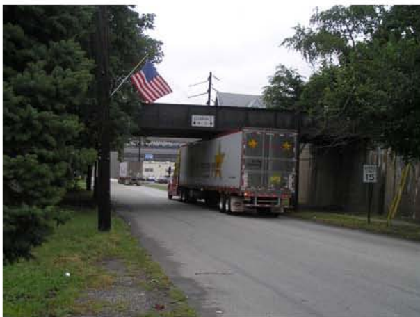
A 14' bridge along the Penn Terminals Connector
