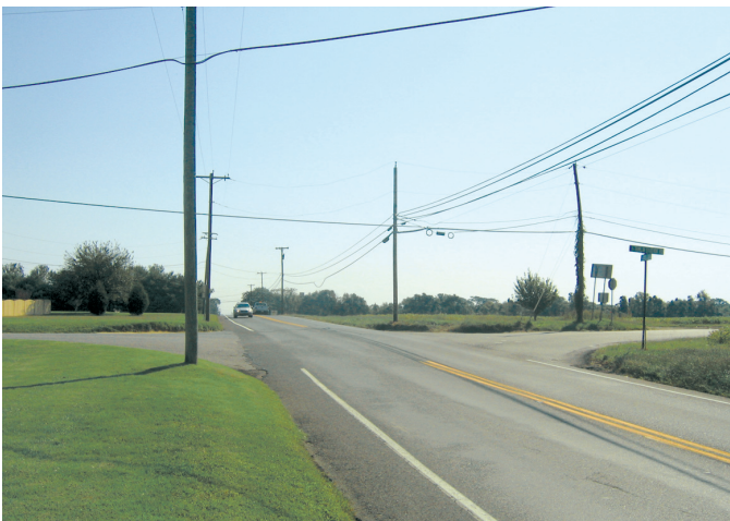
Intersection of US 322 and Tomlin Station Road, Harrison Township
