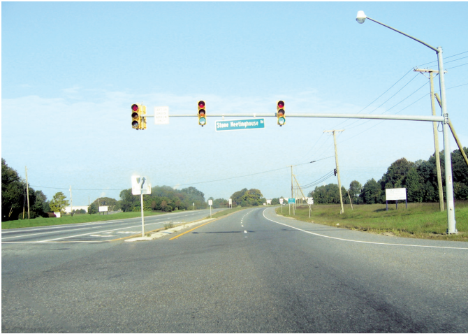
Intersection of US 322 and Stone Meetinghouse Road
