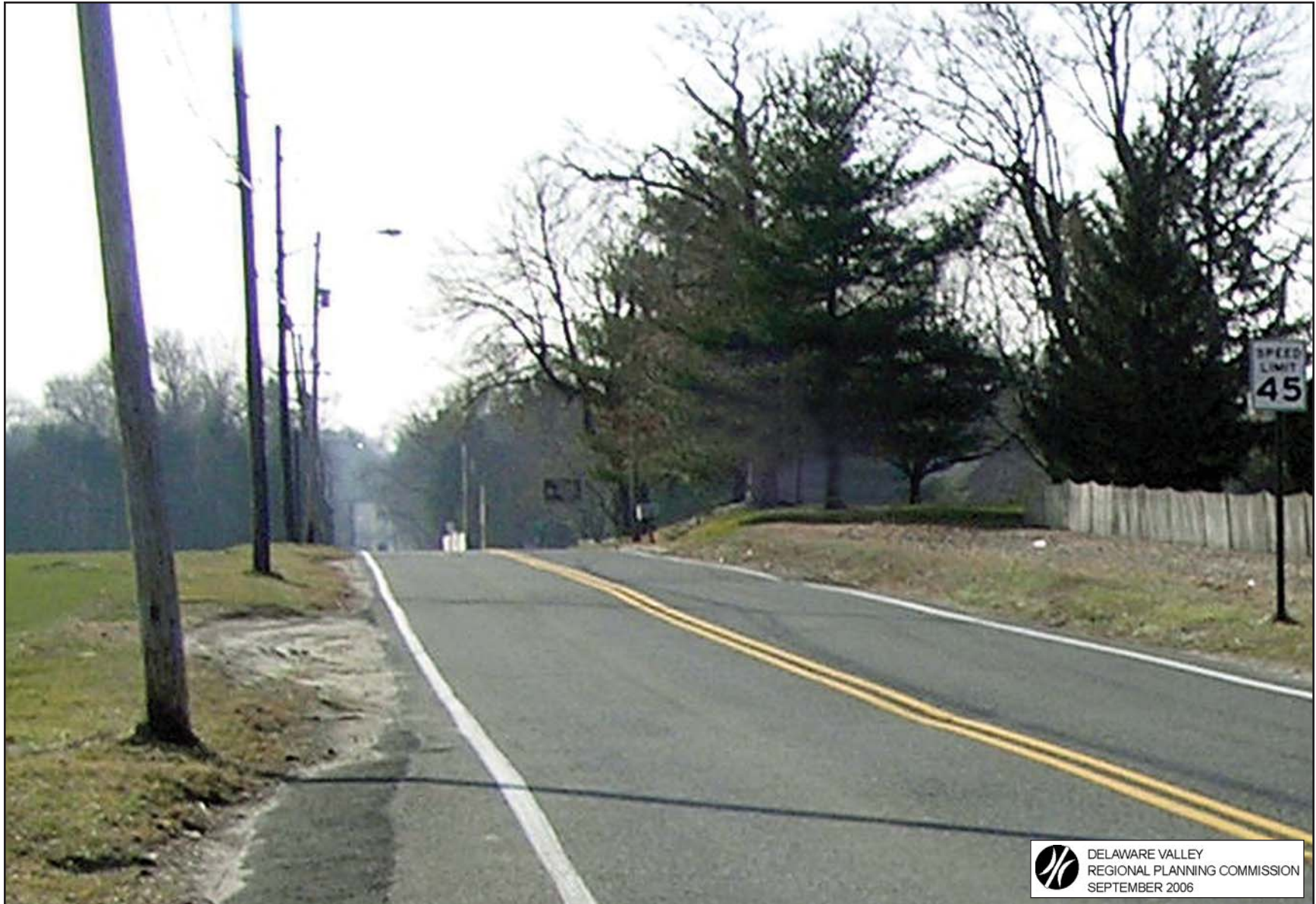
FIGURE 7: Existing conditions along Smithville Road
