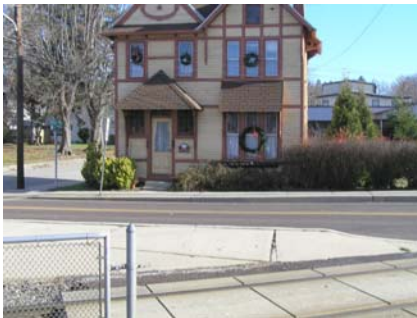
A law office occupies a converted house near the rail line in North Wales.
