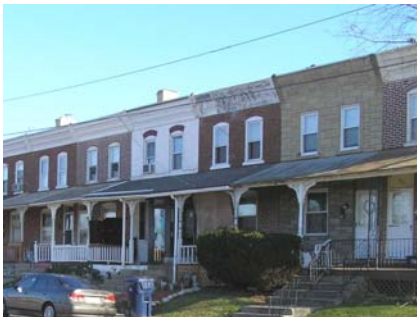
Older row homes located near the Merck complex.
