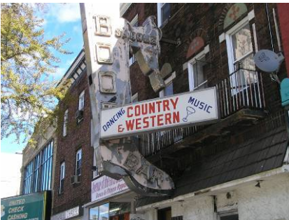
A vacant former country-and-western bar is a development opportunity, given its location next to the subway station. Effort should be made to restore the unique “Boot and Saddle” sign.
