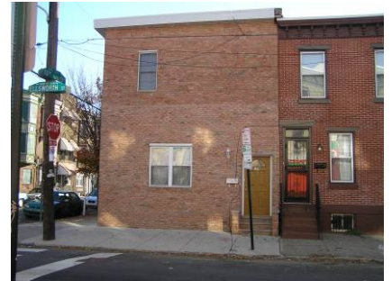
Neighborhood design guidelines or design review might have prevented the removal of the second-story window in this renovation.
