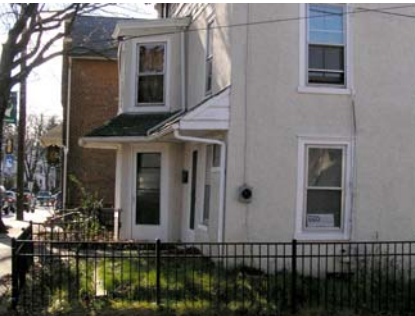
A vacant residential building near North Wales' downtown area.
