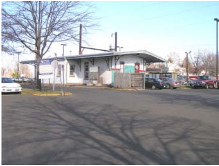
North Wales SEPTA station.
