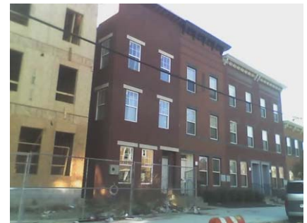
Attractive new infill townhomes are being built where the MLK public housing towers once stood, in the Hawthorne neighborhood, as part of HUD's HOPE VI program.
