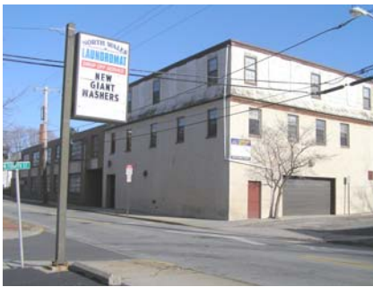
Warehouse property on Walnut Street in downtown North Wales.
