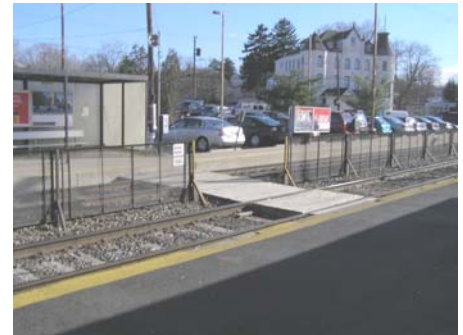
At present, the North Wales station and platform are not fully accessible to individuals in wheelchairs. Construction of planned accessibility improvements is scheduled to begin in 2007.
