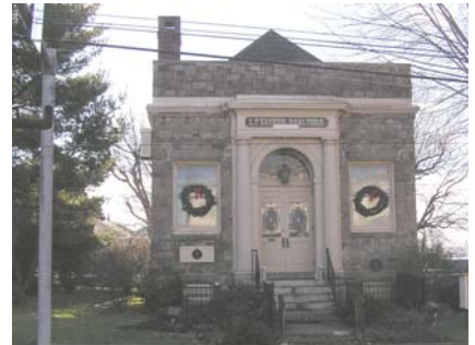
A consignment shop occupies an attractive historic building in North Wales.
