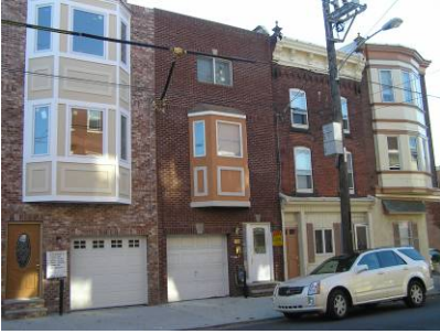
New homes with front-loaded garages detract from the pedestrian experience and remove on-street parking spaces.
