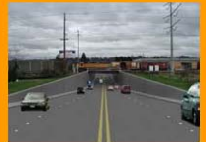
Highway-Rail Grade Separation Kent, WA
