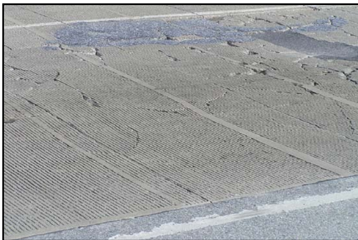
Deteriorated concrete pavement on PA 41
