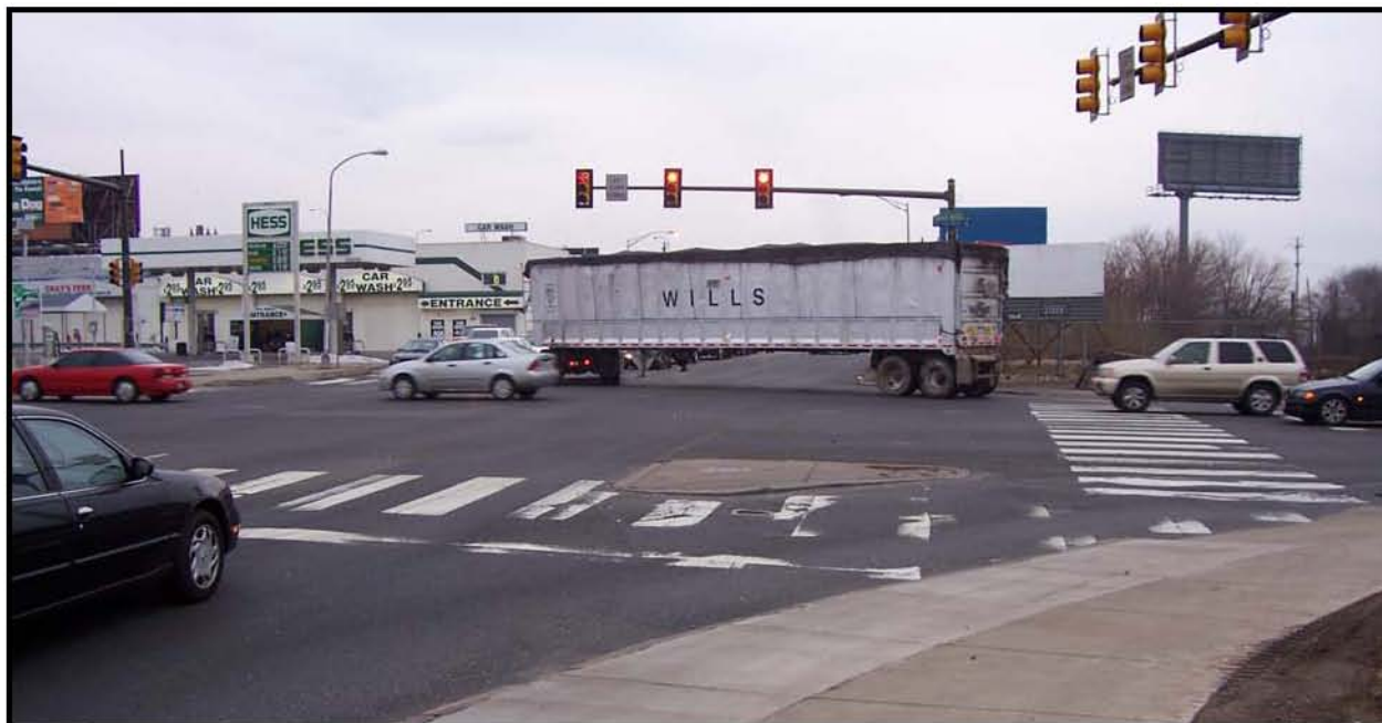
Turning Radius Problem: Tractor trailer making a wide right-turn from Grays Ferry Ave. eastbound to 34 th St. south
