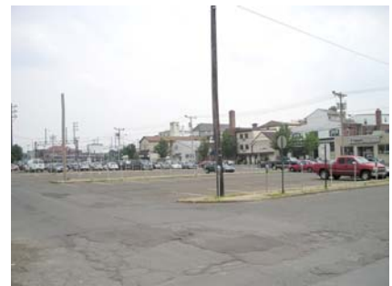
Lansdale’s municipal parking lot is part of the 7.9 acre redevelopment site.
