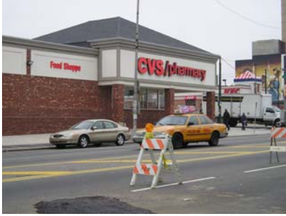
New CVS at Broad and Girard is built to the street line.
