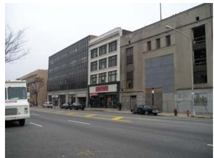
Vacant art deco building, next to laundromat, hair salon, OIC, and Sneaker Villa on North Broad Street.
