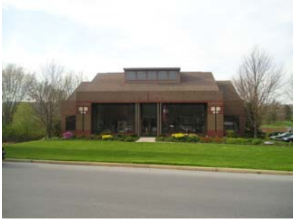
Thorndale Dental Associates on C.G. Zinn Road is an attractive new building north of the station. Sidewalks could help connect this area to the station.
