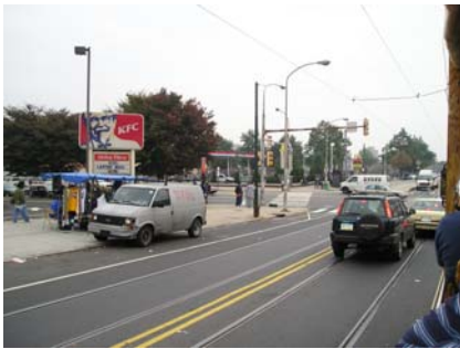
Narrower roadway along 1400 block of Girard necessitates a street-running trolley.
