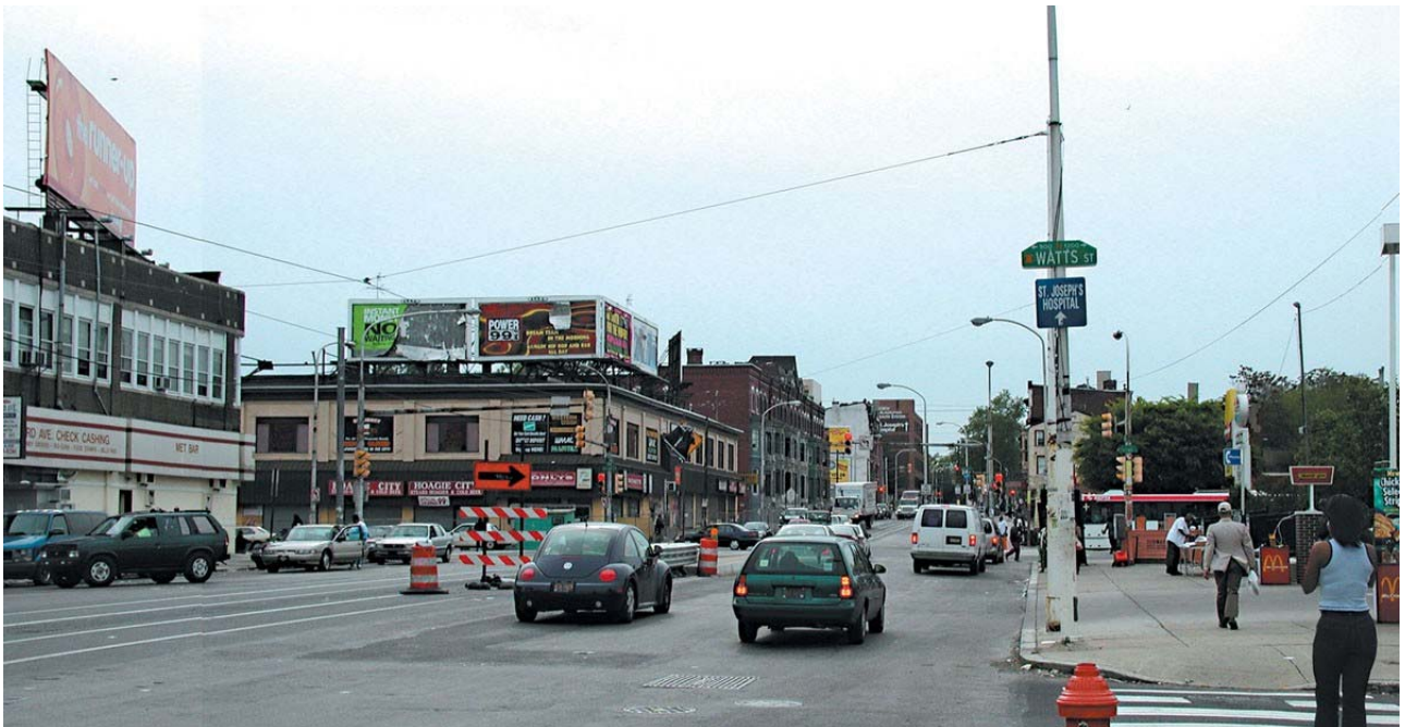
Figure 3: Girard Before Photograph shows the intersection of Broad and Girard streets before the CVS was built last year.
