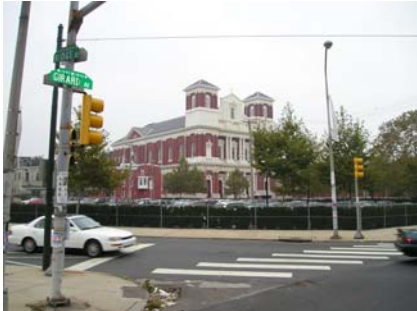
Church of the Gesu next to St. Joseph’s Preparatory School on Girard Avenue.
