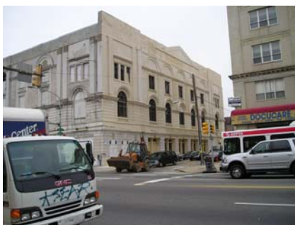
North side of Metropolitan Opera House, under renovation.
