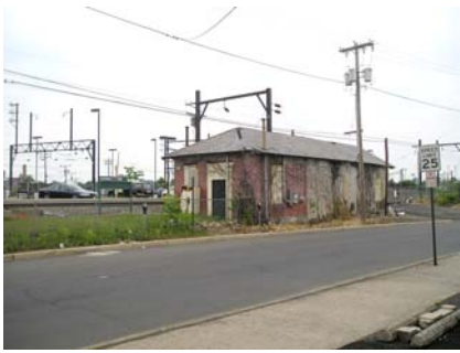
Utility building located near station and large redevelopment site.
