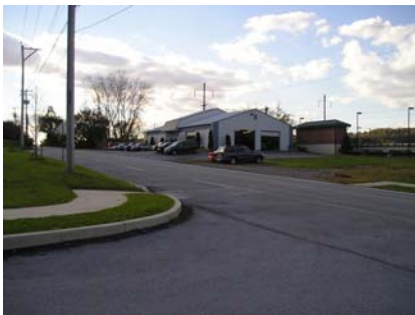
South Bailey Road is the main access road to the south of the station, though it lacks continuous sidewalks and transit-friendly uses. Pictured above is the Dupont Auto Body Shop.
