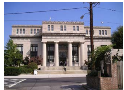
Woodbury is the county seat and is home to many fine buildings, such as the Gloucester County Building.
