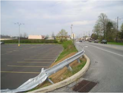
There are very few sidewalks along U.S. Route 30.
