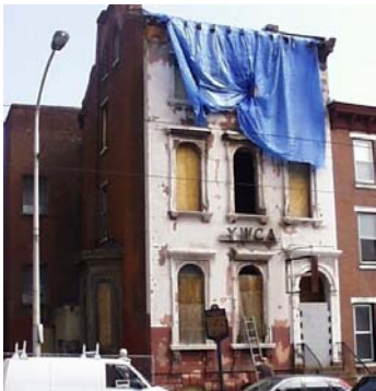
YMCA under renovation on 1500 block of Girard.
