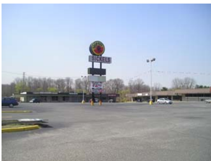
The Sickel's Shopping Center adjacent to the South Barber site is a redevelopment opportunity.
