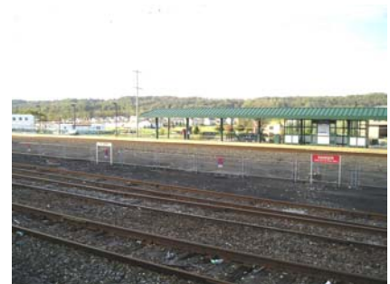
SEPTA and Amtrak trains run along these tracks in Thorndale. SEPTA Cross County Metro trains could join them in the future.
