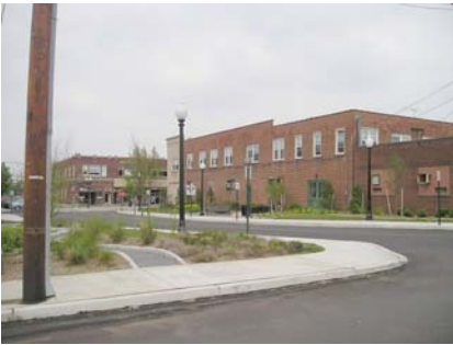
Apartments above and behind stores on Main Street.
